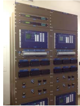
Rack with PMUs in a BPA substation
