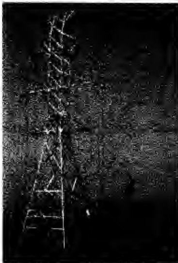
This new double-circuit 500-kilovolt tower is put to the test at a facility in India. To see if it
