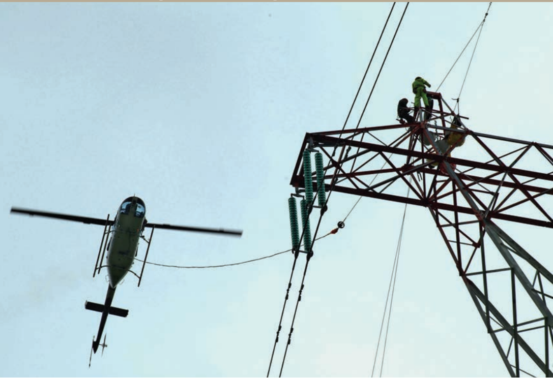
Using precision flying techniques, a BPA helicopter pilot helps crews string fiber optic cable.
