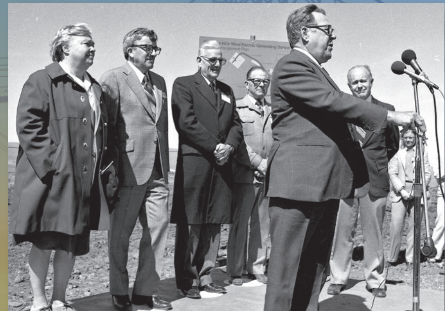
Washington Sen. Warren Magnuson is joined by Gov. Dixy Lee Ray (left), Boeing CEO Thornton "T" A. Wilson (dark overcoat) and BPA Administrator Sterling Munro (right) at Goodnoe Hills for the 1980 groundbreaking ceremony for the world's first multimegawatt, commercially viable wind farm. The project, called the MOD-2, was undertaken by USDOE, NASA, Boeing, Battelle, Klickitat County PUD and BPA.
