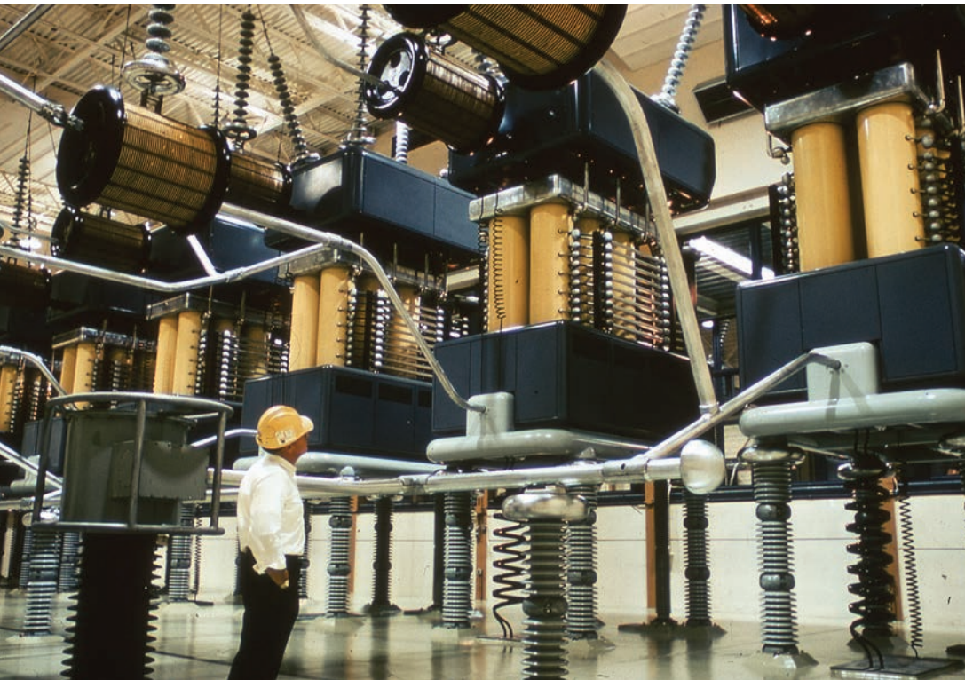
The 1970s construction of BPA's Celilo Converter Station included mercury-filled power converters, above. In 1985, BPA installed new semiconductor-based switches, right, boosting the direct-current line's capacity from 1,600 megawatts to 2,000 MW.
