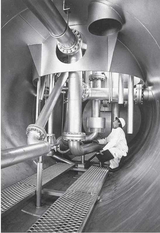
Decommissioning of mothballed nuclear power plant WNP-1, which was never completed, began in 1995.
