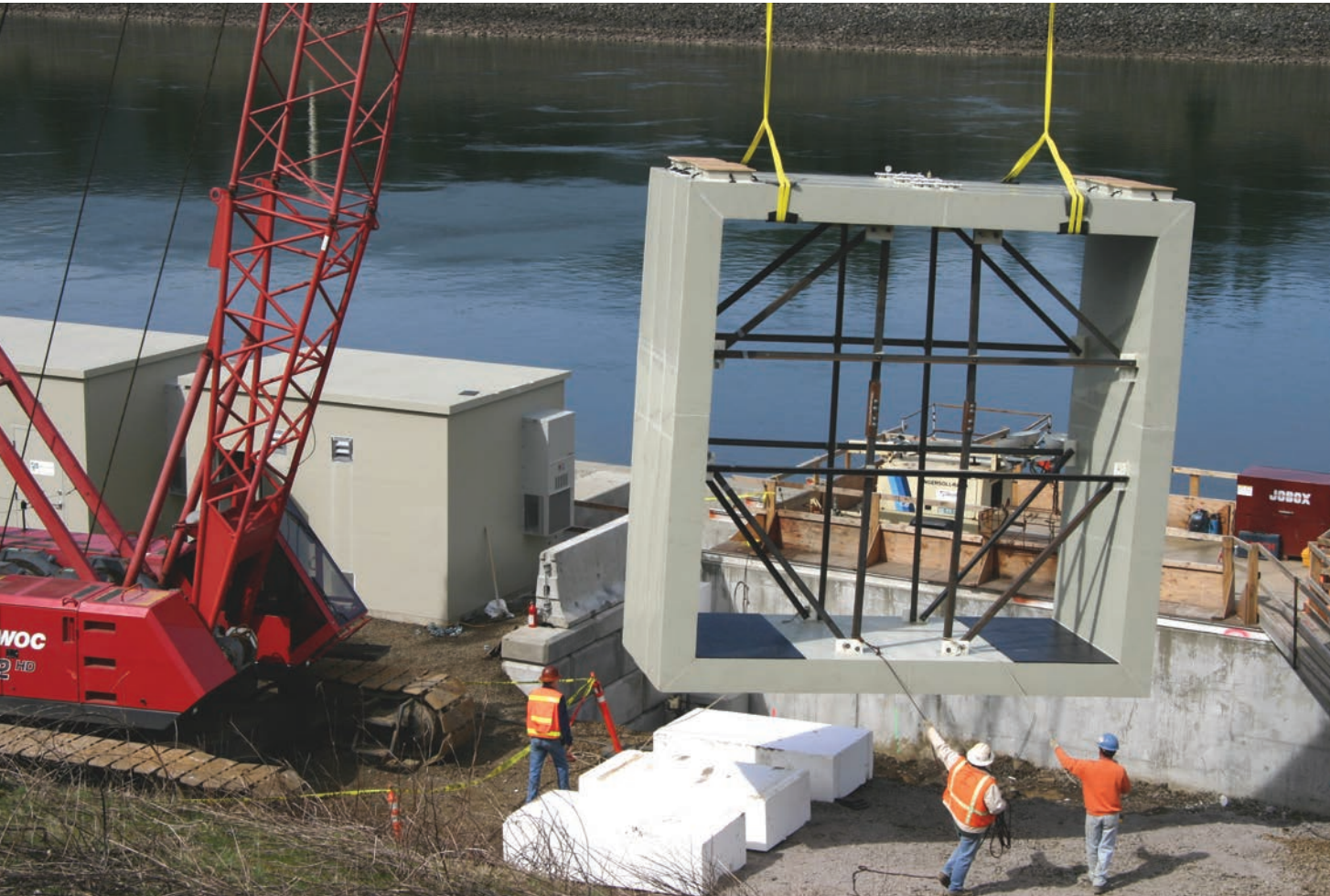
In 2006, workers lower a square PIT-tag antenna, the largest of its kind in the world, into the outlet flume from the Bonneville Dam corner collector, the dam's surface passage system for juvenile fish. (Scott Bettin/BPA)
