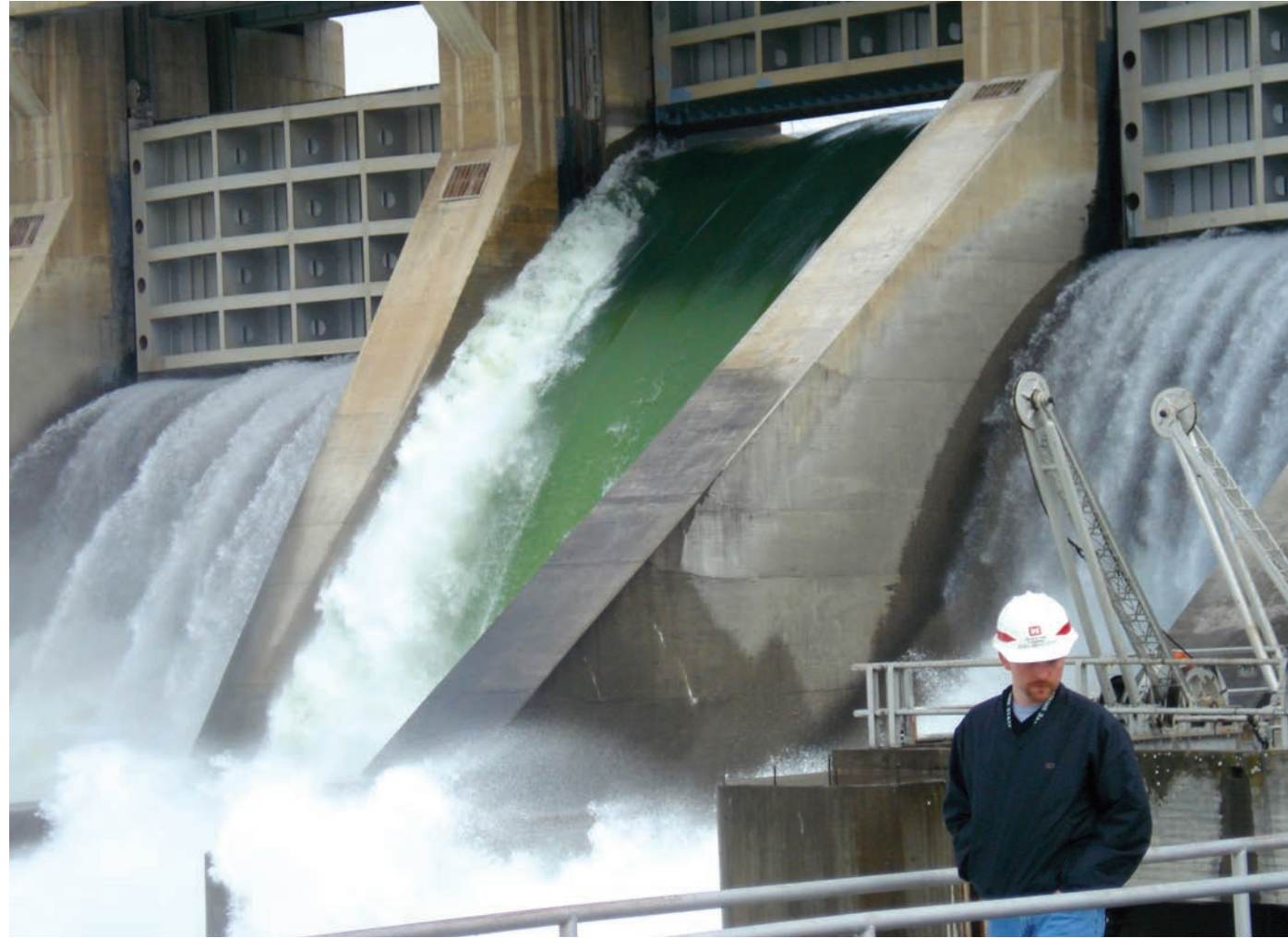
Water rushes over a spillway weir at McNary Dam, easing the downstream migration for juvenile salmon and steelhead by providing passage at the river’s surface — where they naturally migrate. (Scott Bettin/BPA)
