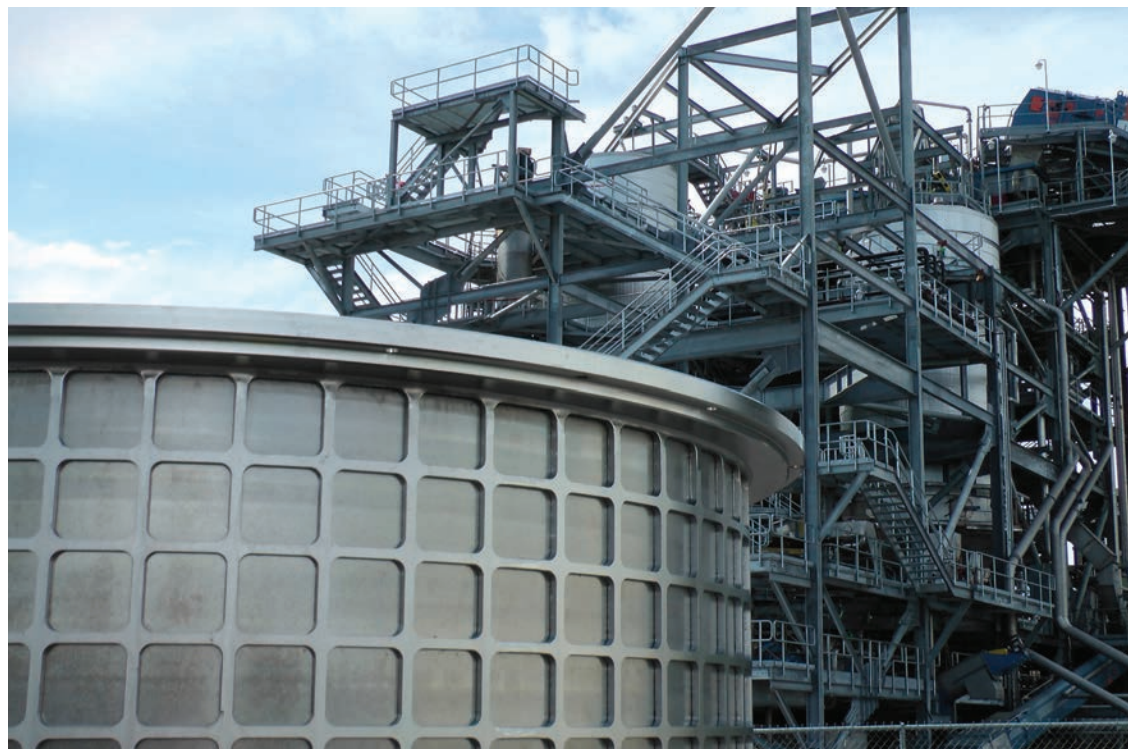
A pretreatment structure for wood chips at NORPAC, the continent’s biggest newsprint producer, is part of the largest energy efficiency project in the Northwest and one of the largest in the country. In 2012, BPA and Cowlitz County Public Utility District partnered with North Pacific Paper Corp., owner of the Longview, Wash., paper mill, to reduce the electricity and chemicals needed to refine wood chips, saving enough energy to serve 8,000 Northwest homes. (Brent Arnold/Cowlitz County PUD)
