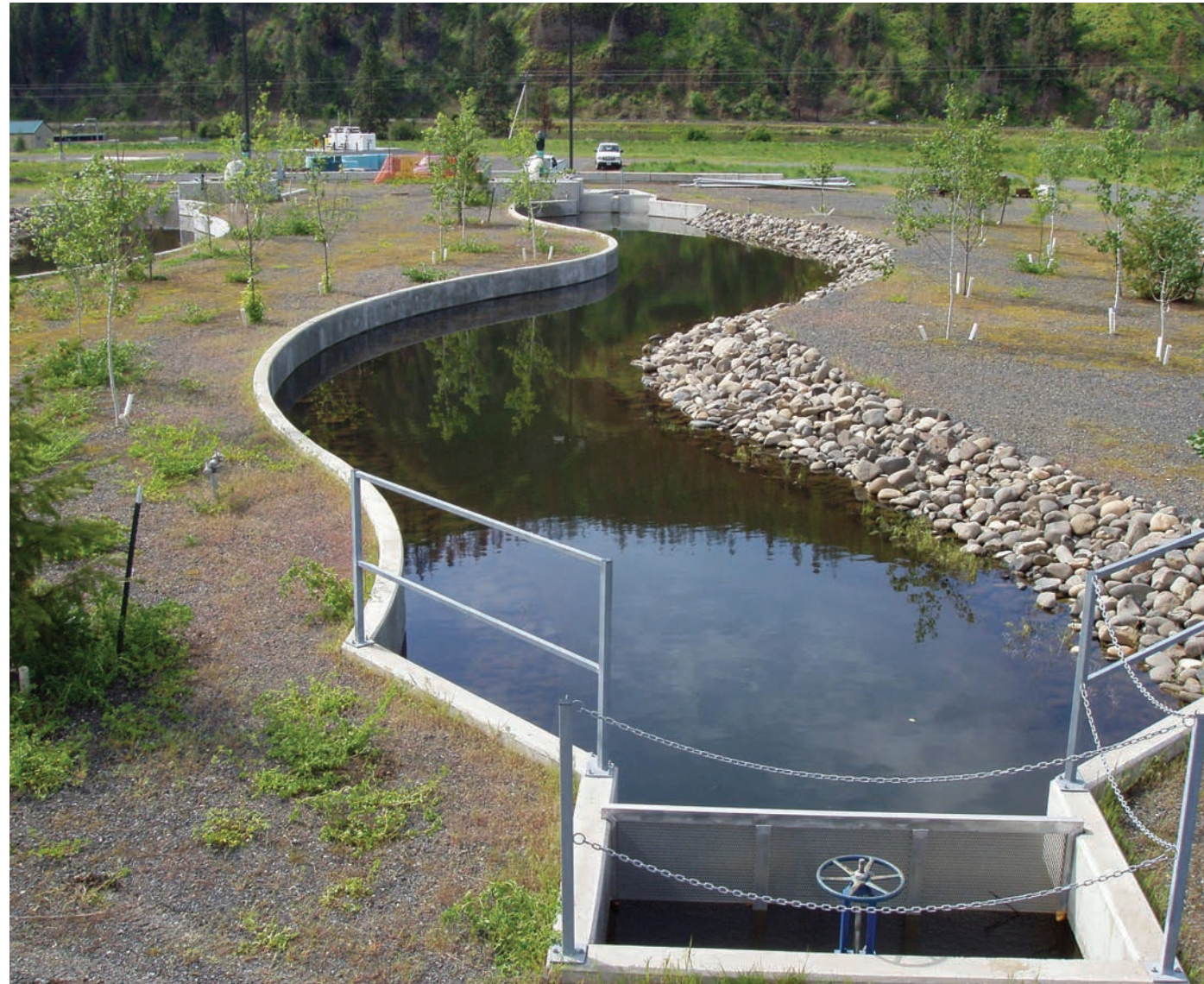
Sinuous raceways at the Nez Perce Tribal Fish Hatchery mimic the curves of natural rivers and streams so fish raised at the hatchery are better prepared for life in the wild. (Jonathan McCloud/BPA)
