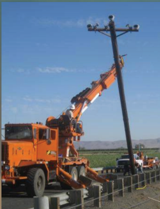
An all Native American line crew from Yakama Power replaces a damaged power line in June 2011 with a truck on loan from BPA. The Yakama Nation formed its own utility, with assistance from BPA, and began purchasing power to serve members near Toppenish, Wash., in 2009. (Yakama Power)
