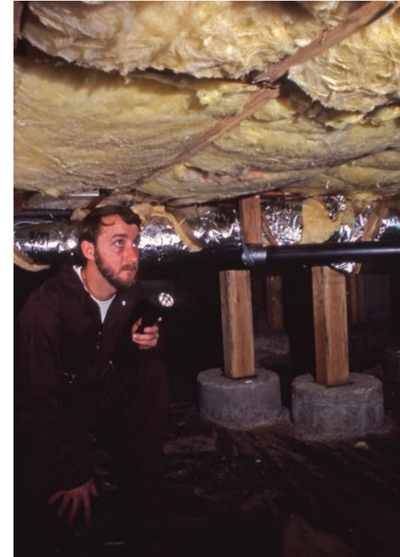
BPA engineers peered into crawlspaces to inspect insulation jobs for the weatherization program.
