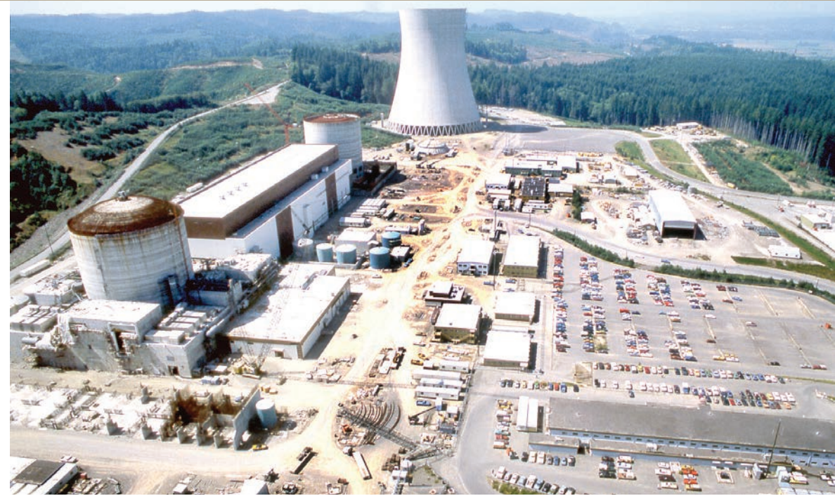
Construction began on WNP-3 and WNP-5 but was never completed. BPA Administrator Peter T. Johnson declared WNP-3 must be mothballed and the WPPSS board adopted a resolution terminating WNP-1 and -3 May 13, 1984.
