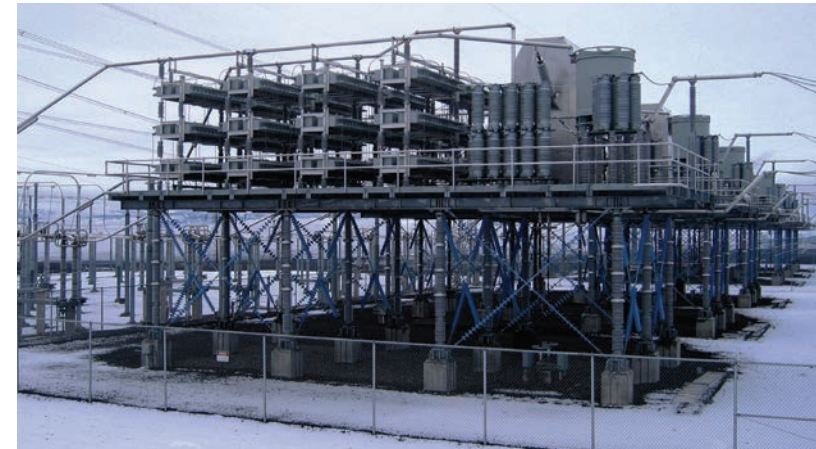
Series compensation devices, such as these at BPA's Schultz Substation, store voltage momentarily. Huge banks of them along lengthy transmission lines help keep the power system stable.
