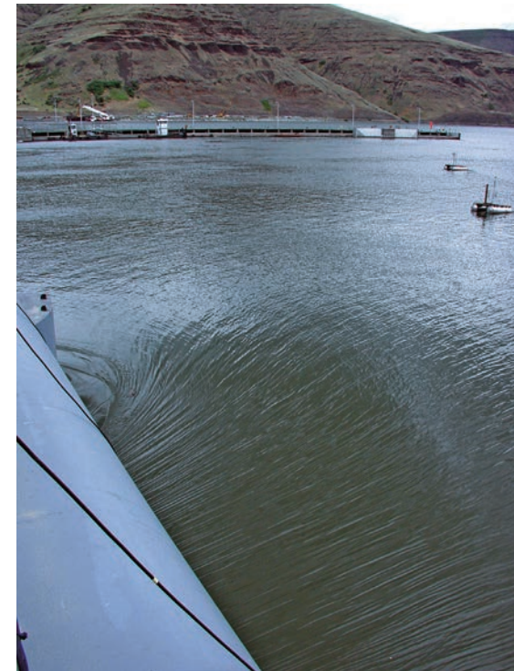
Water from the surface of the Snake River swirls over a spillway weir at Lower Granite Dam. (Scott Bettin/BPA)
