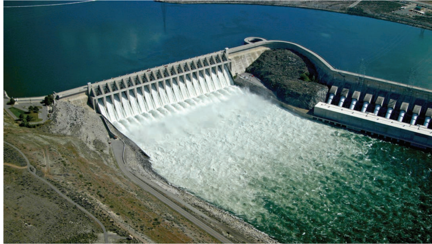
The Corps of Engineers completed flow deflectors at Chief Joseph Dam in 2009. The deflectors send streams of water upward at the base of the dam to help dissolved gas dissipate so it does not harm fish. (Scott Bettin/BPA)
