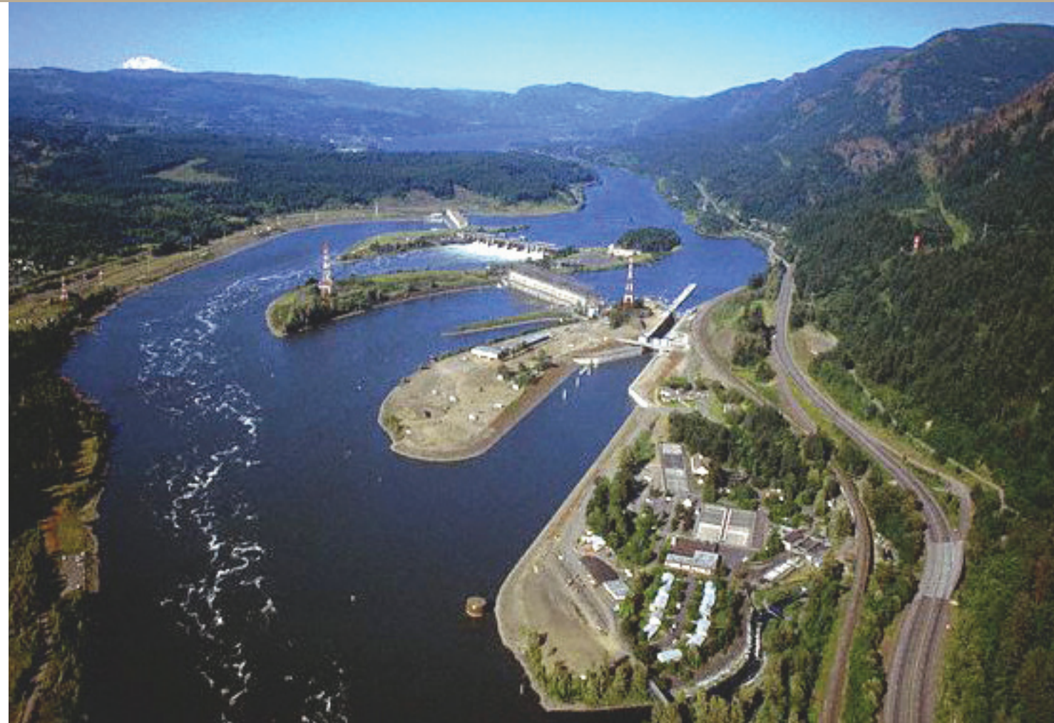
Bonneville Dam, the first federal dam constructed on the Columbia River, was completed by the U.S. Army Corps of Engineers in 1937, the same year the Bonneville Power Administration was created. An Oregon Department of Fish and Wildlife hatchery is in the lower right foreground. (Philip James Corwin/Corbis)
