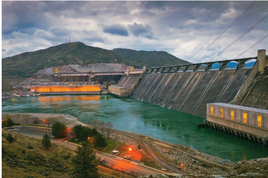
Grand Coulee Dam is the largest power plant of any kind in the United States. The dam's generating capacity of about 7,000 megawatts is nearly double that of the next largest power plant, according to the Energy Information Administration. (© Gary Weathers/Tetra Images/Corbis)
