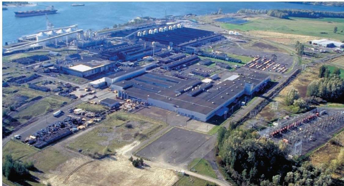
Alcoa's Vancouver, Wash., aluminum smelter, built in 1940, was the first to use power from the Columbia River. It operated until a 1986 labor dispute. Private investors bought the plant in 1987 and operated it as Vanalco until the West Coast power crisis in 2000.
