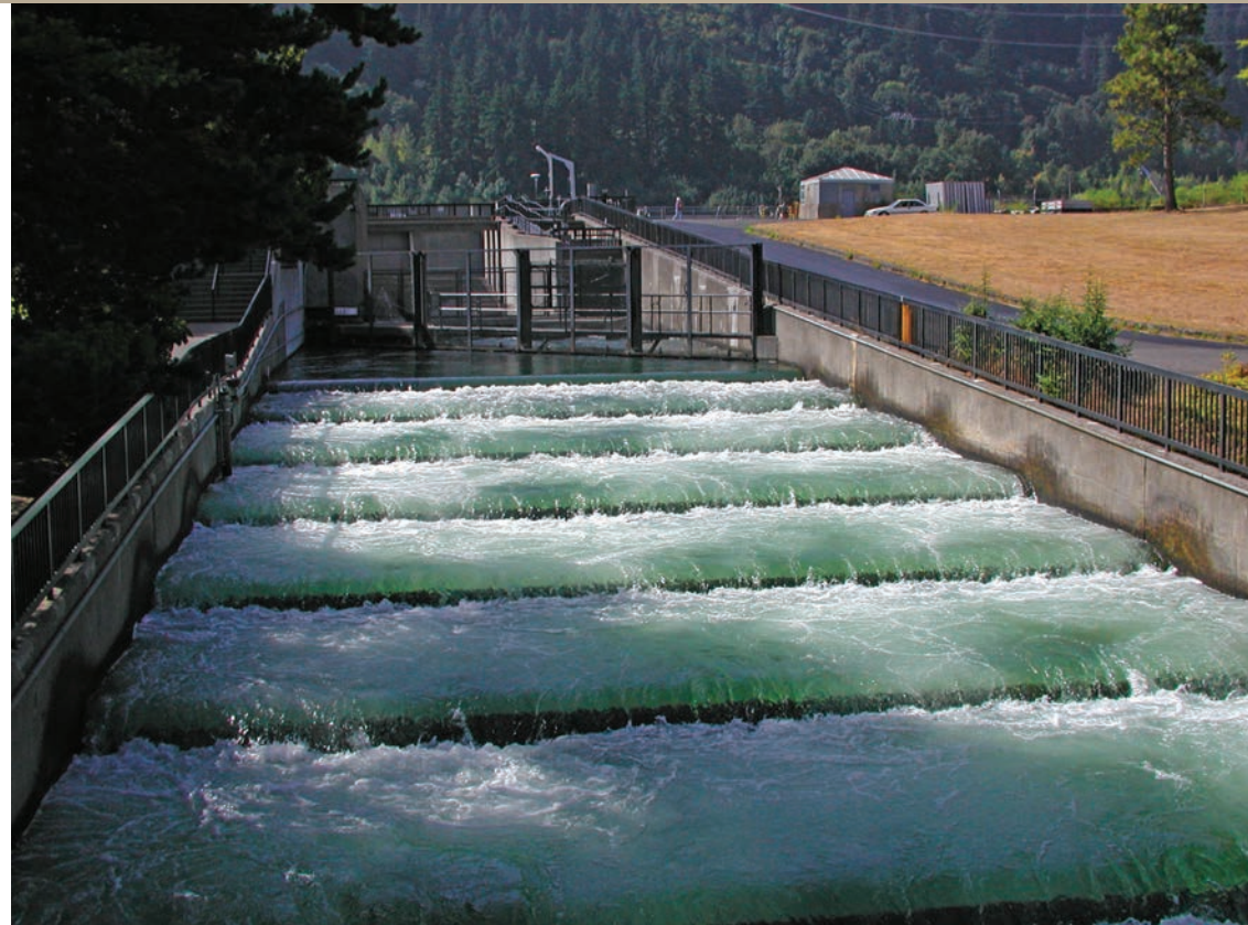
Fish ladder at Bonneville Dam.
