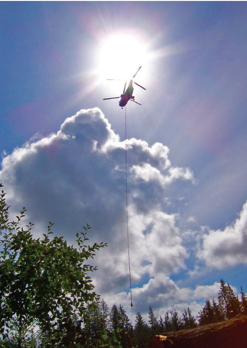
A helicopter lifts tower sections into place on the Kangley-Echo Lake line to minimize impacts on the ground.
