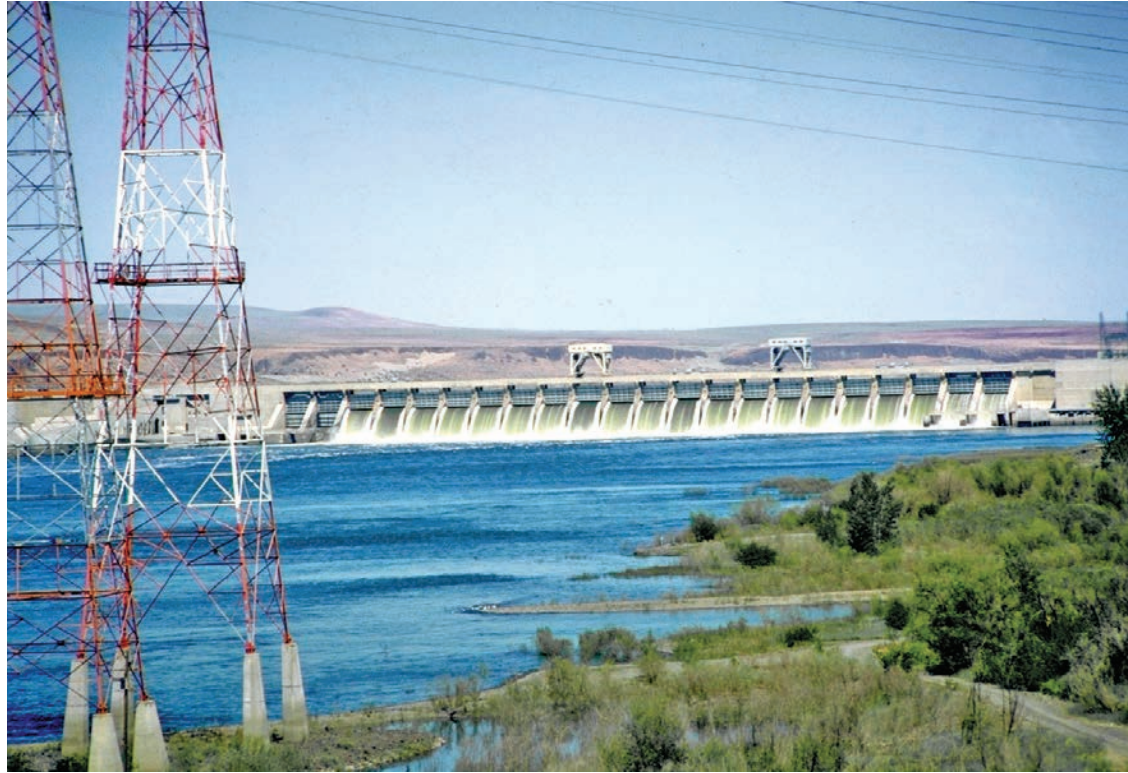
McNary Dam, near the head of the intertie, provides critical voltage support for the lines to California. But cascading line outages in 1996 strained the transmission system and caused the dam to trip off line. It was the final blow in a catastrophic series of events.
