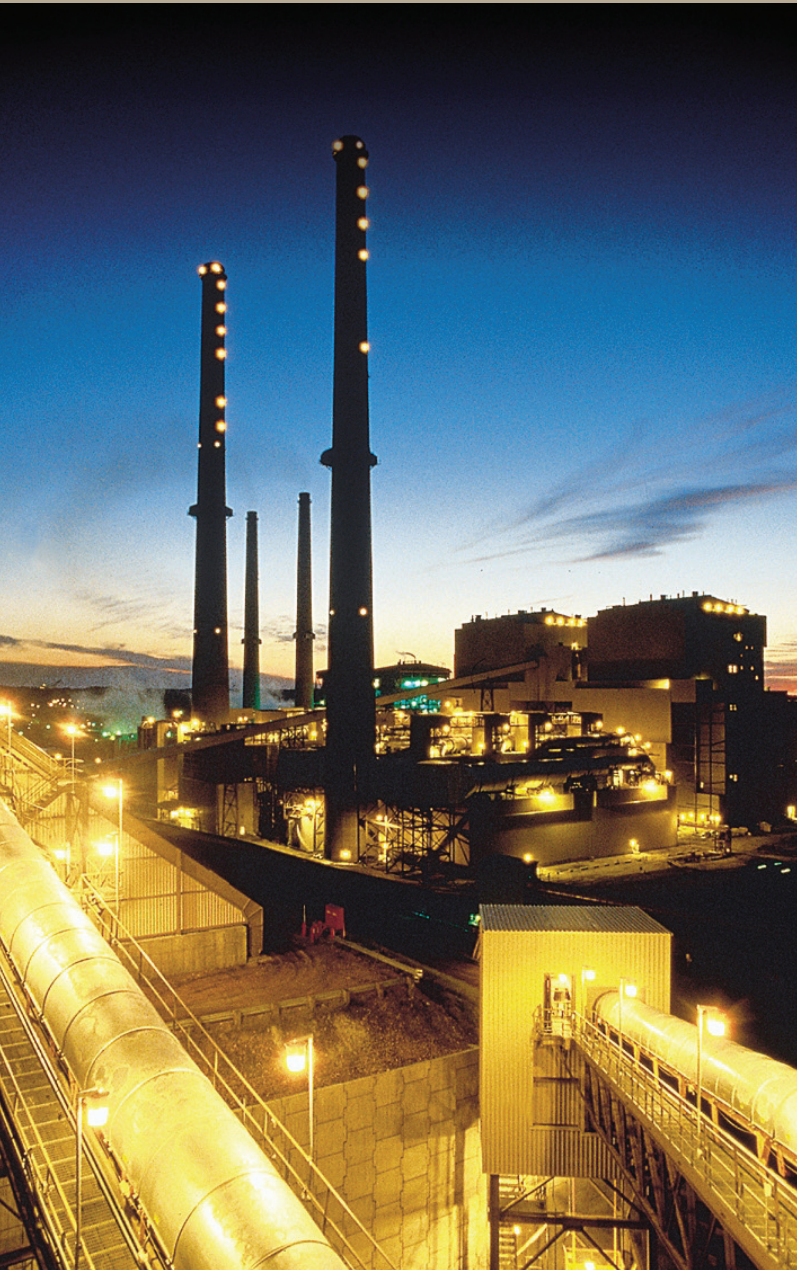
The Colstrip coal-fired power plant was already under construction when BPA agreed to build the new line. Utilities had invested millions of dollars, and the agency faced intense pressure to build the line quickly. (PPL Corp.)
