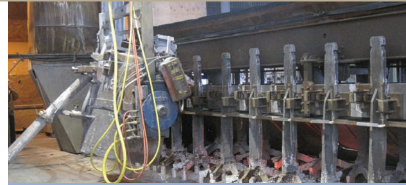
Aluminum potlines, used to smelt ore into aluminum, were a key area for efficiency improvements in ConMod.
