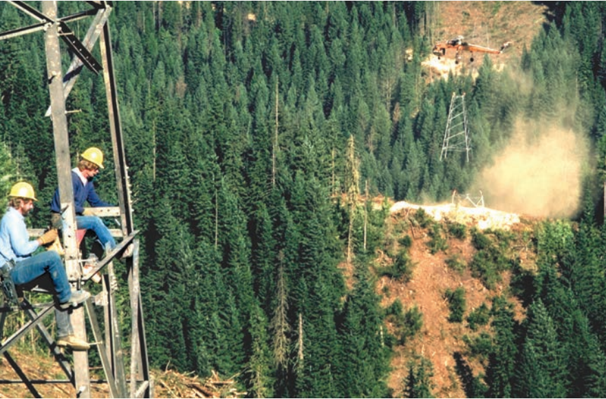
Helicopters flew equipment into the rough Montana terrain, speeding construction.
