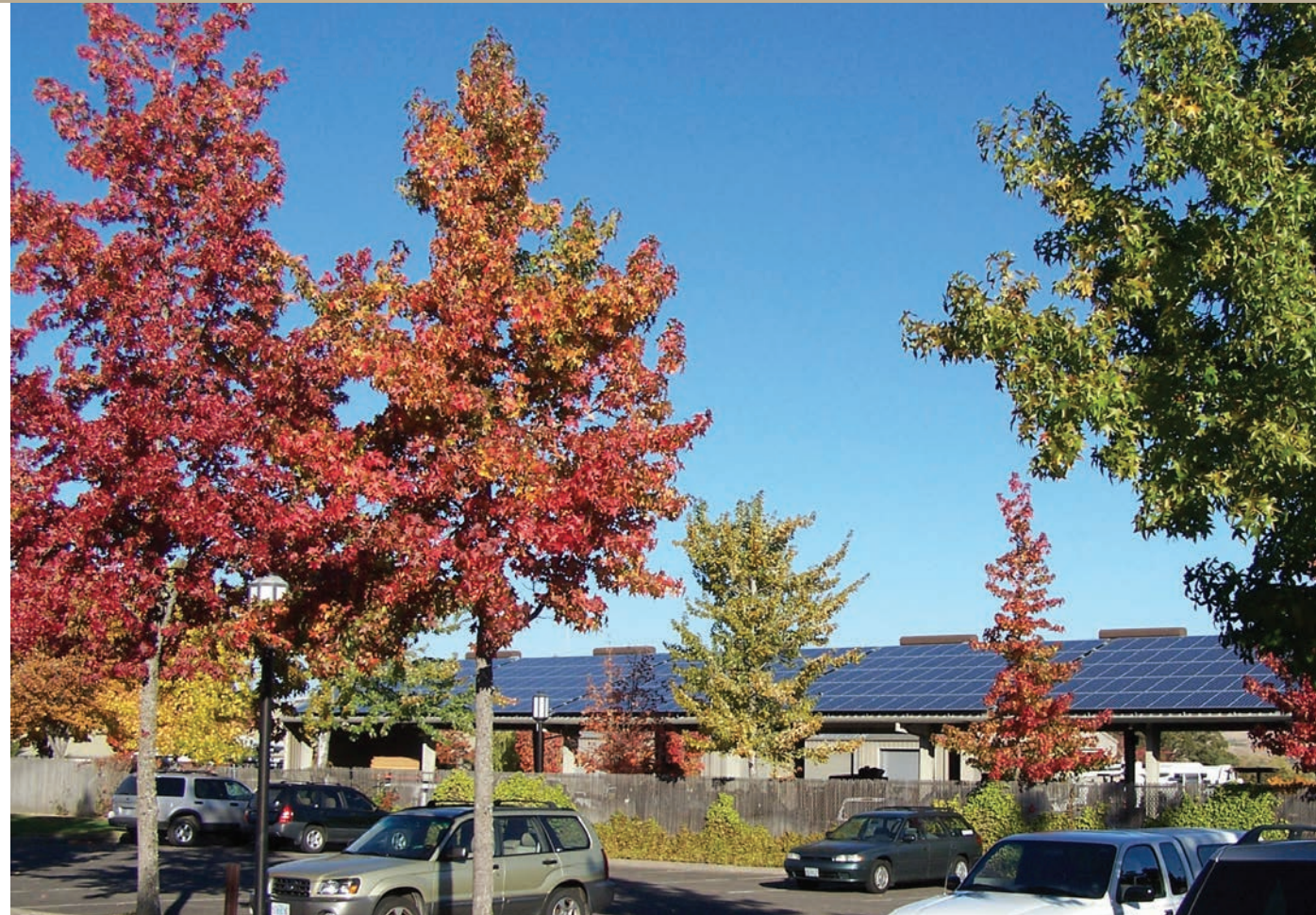
In 2008, the City of Ashland, Ore., installed 363 photovoltaic panels on a city utility vehicle parking structure. Consumers who purchase shares of the 64 kilowatt “Community Solar” project receive credits on their utility bills for electricity that the project generates.
