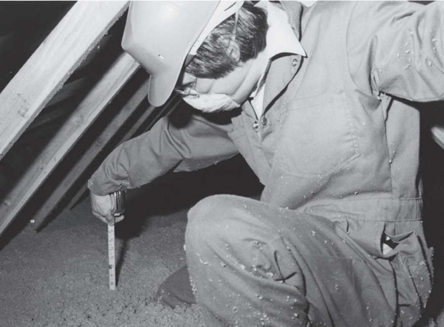
BPA's weatherization specifications called for attic insulation depths of 12 inches or more.
