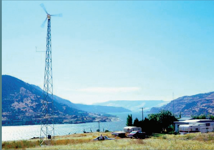
Construction of the MOD-2 wind turbine cluster began in 1980, and the project's three experimental 2.5-MW generators were brought on line over the next two years. (Rod Aho/BPA)
