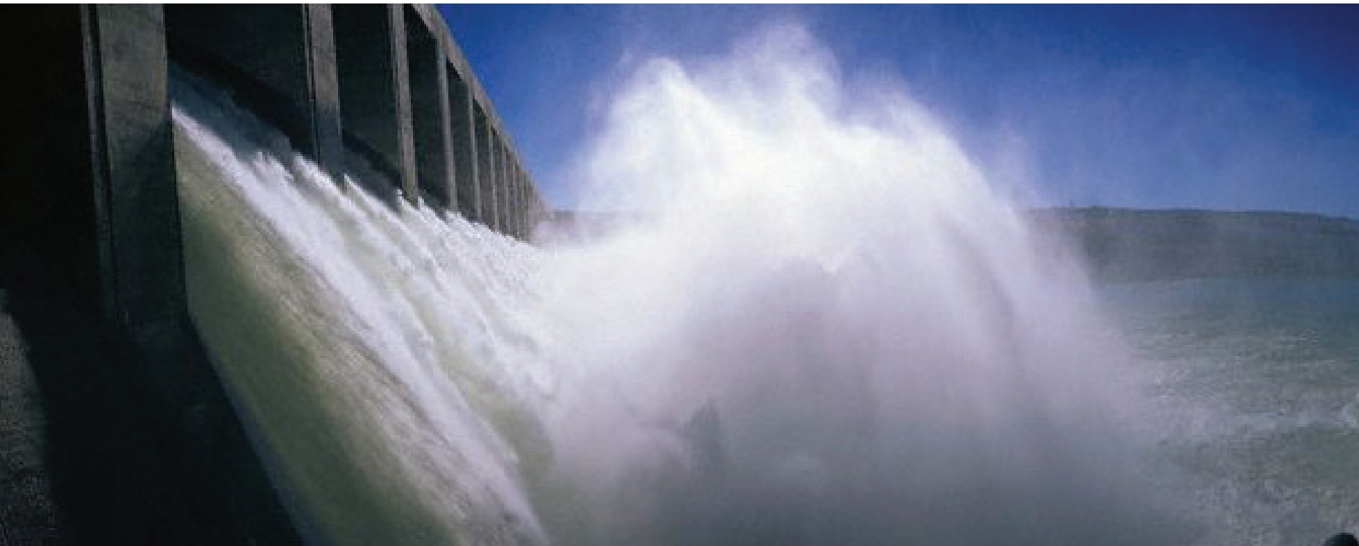
Spray rises from the spillways at Chief Joseph Dam.
