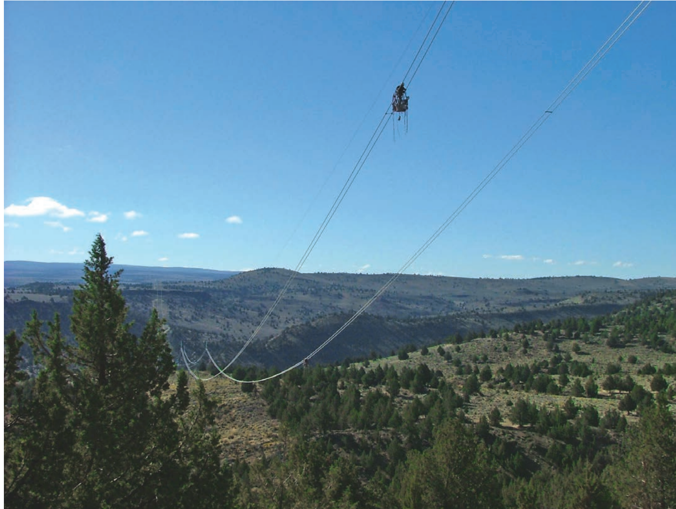
BPA line crews maintain transmission lines through rough and often scenic terrain.
