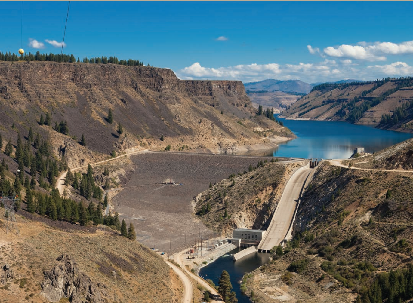
Anderson Ranch Dam on the South Fork of the Boise River north of Mountain Home, Idaho, is one of the smaller dams in the federal system. Its two generating units were updated in 1986 to a combined capacity of 40 megawatts.
