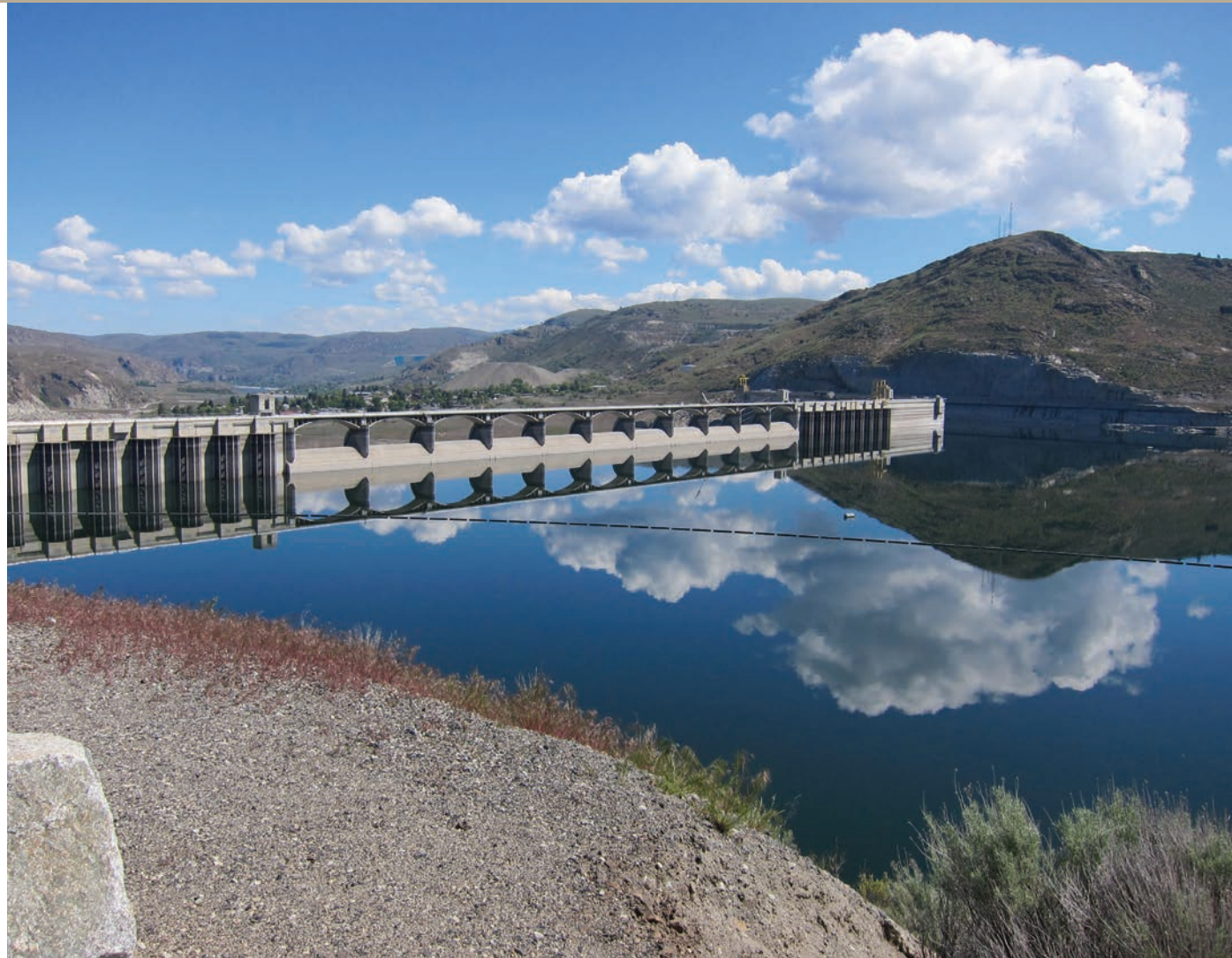
Lake Roosevelt stands mirror smooth behind Grand Coulee Dam, the largest source of power generation in the Columbia River hydroelectric system. (Geri Campbell/BPA)
