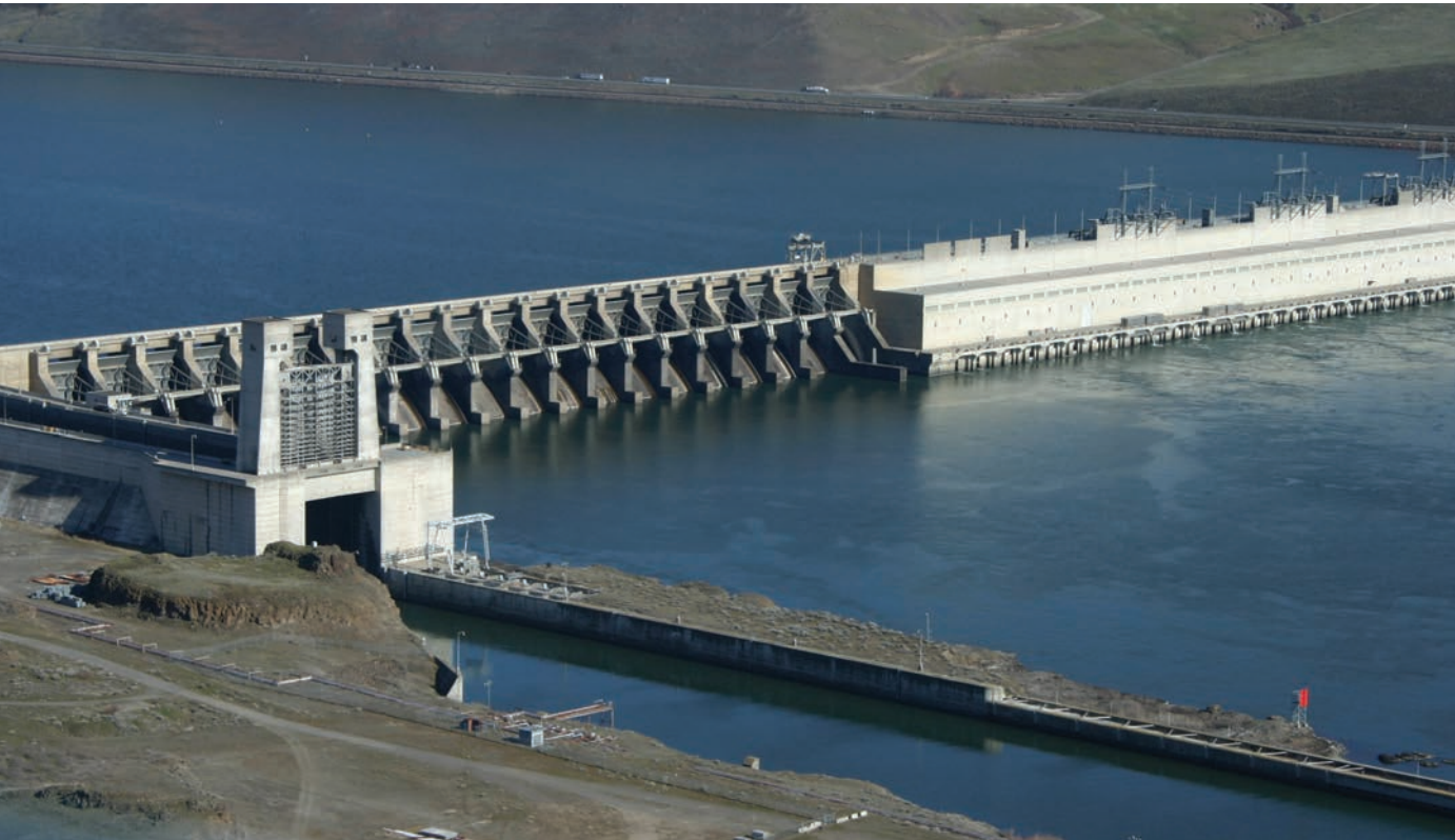
Spillways stand empty at John Day Dam while available water turns turbines.
