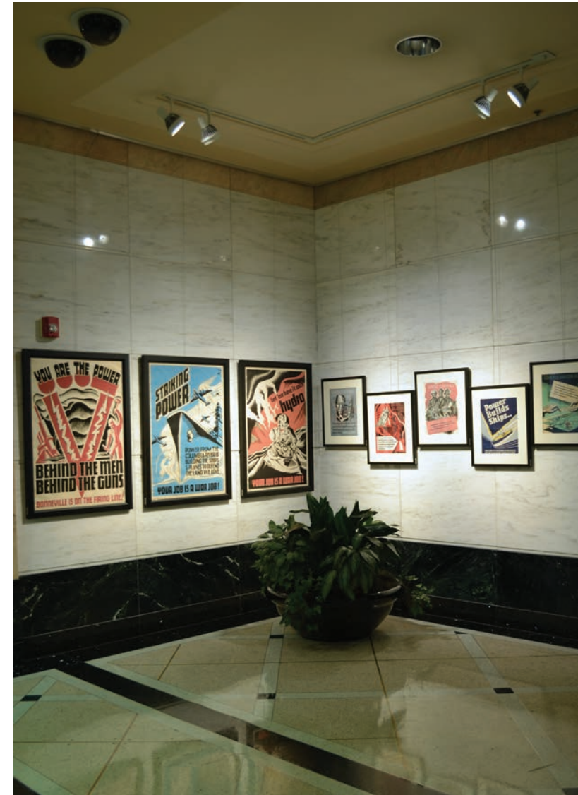
LEDs (light-emitting diodes), installed in the BPA headquarters lobby in 2010, use about 25 percent less energy than compact fluorescent bulbs and illuminate the artwork more effectively. BPA is pilot testing new uses for LEDs and expects their practical application to grow over the next decade.
