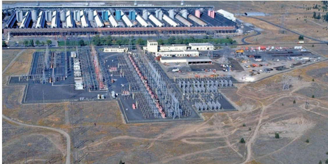
Kaiser Aluminum plant near Spokane, Wash., with BPA's Bell Substation in the foreground.
