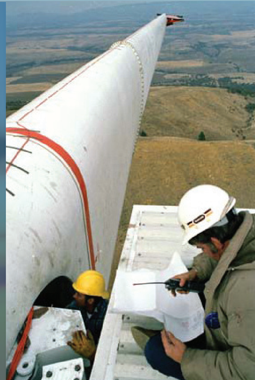
Technicians fine tune mechanisms inside a MOD-2 wind turbine. At 200 feet above ground, the generating units required a crane to move heavy pieces of equipment. (NASA)
