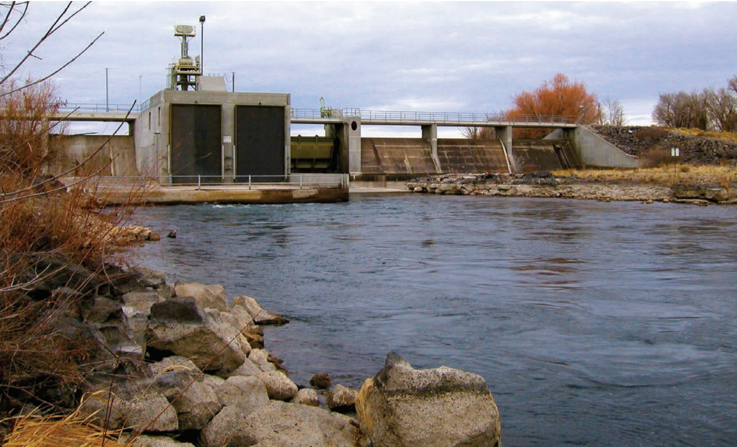
BPA's first resource acquisition under the Northwest Power Act was the output of a City of Idaho Falls hydroelectric project called the Bulb Turbine Project on the Snake River. (Kevin Getsinger/Idaho Falls Power)
