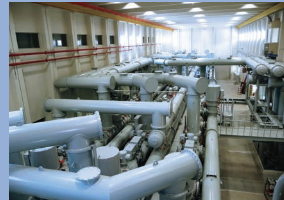
Squeezing a 15-acre substation into a 60-by-200-foot building keeps Taft Substation operating despite snow that can be 10 feet deep in a typical winter.
