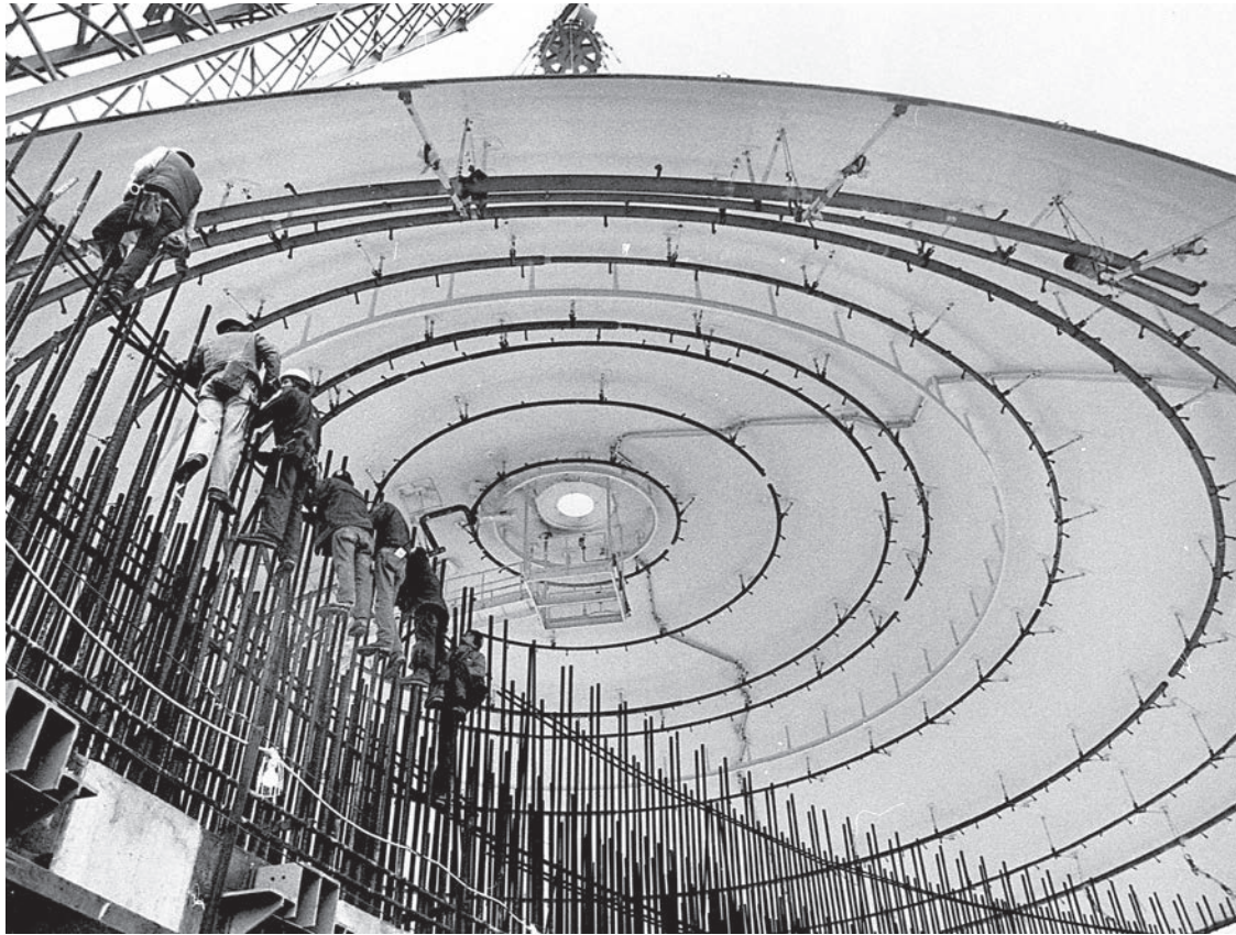
Construction continues on WNP-3, providing employment for thousands of workers.
