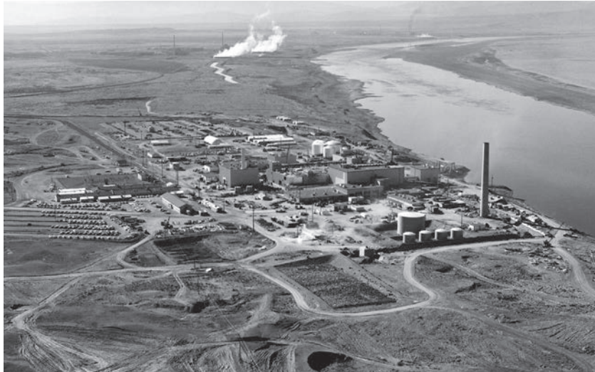
Hanford's N Reactor is called a dual-purpose reactor because it not only produced plutonium for America's defense program, but also generated electricity marketed by BPA. At construction in the early 1960s, it was the only reactor of its kind in the nation.
