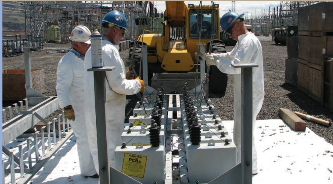
A rigging crew packages capacitors containing PCBs for disposal. The BPA crew, in blue hard hats, includes (from left) Walt Finney, Tom Wellman and (in the cab) Tom Thomas.
