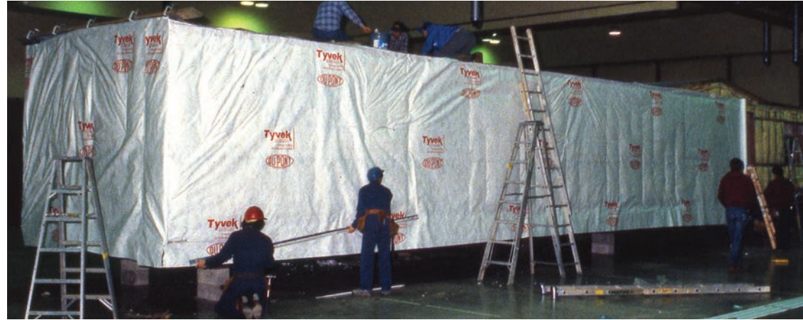
A manufactured home gets wrapped with insulation in the factory, before it's delivered to the lot or the home buyer. BPA worked with utilities and manufacturers to get 100 percent of all manufactured homes sited in the Northwest built to Super Good Cents efficiency standards.
