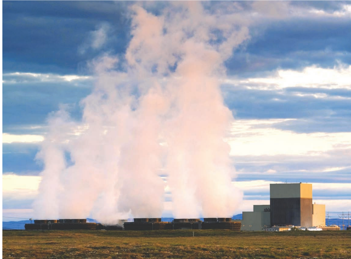
BPA funds and markets the power from the Columbia Generating Station, originally called WNP-2. The plant’s reliable and emission-free power complements the federal hydroelectric system.
