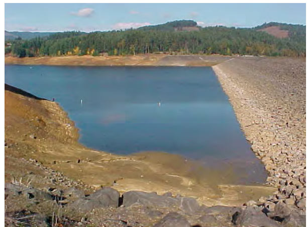
Photo 3-1. Scoggins Dam at low pool (October 2001).
