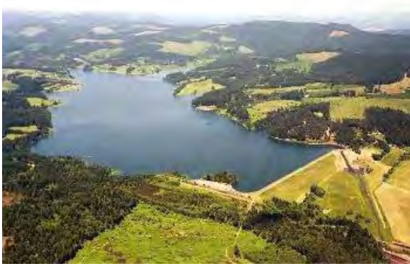
Photo 1-1. Aerial view of Scoggins Dam, Henry Hagg Lake, and surrounding area.
