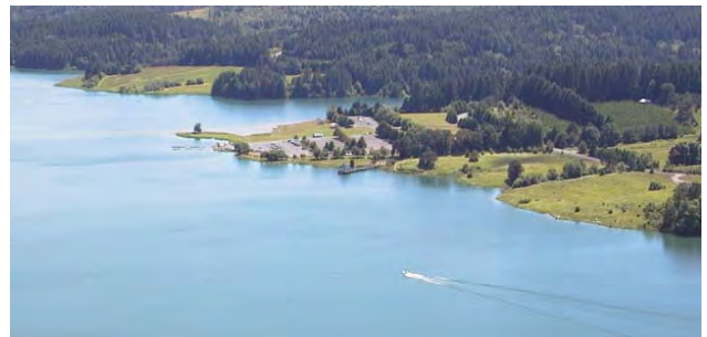
Photo 3-3. Aerial view of Recreation Area C (center) and adjacent Cove Area (right).
