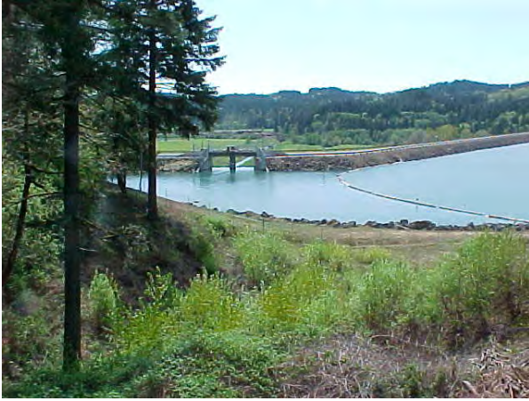
Photo 1-2. Scoggins Dam and spillway at full pool.
