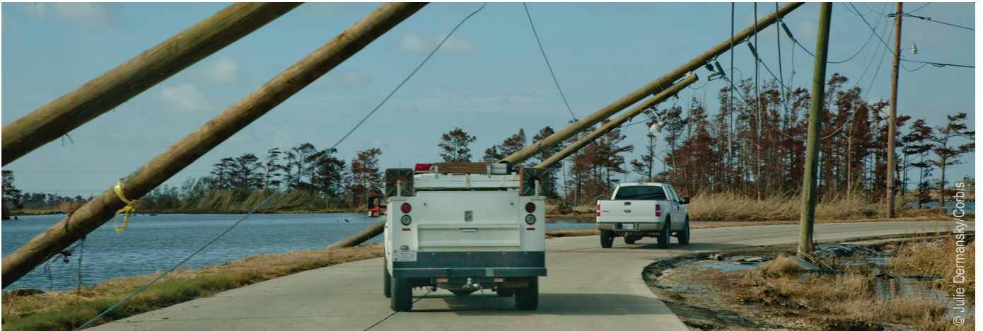
(Top) A truck gets stuck in the storm surge covering Highway 90 in Gulfport, Mississippi, during Hurricane Isaac. (Bottom) Power lines damaged in Plaquemines Parish, Louisiana, by Hurricane Isaac. September 3, 2012.
