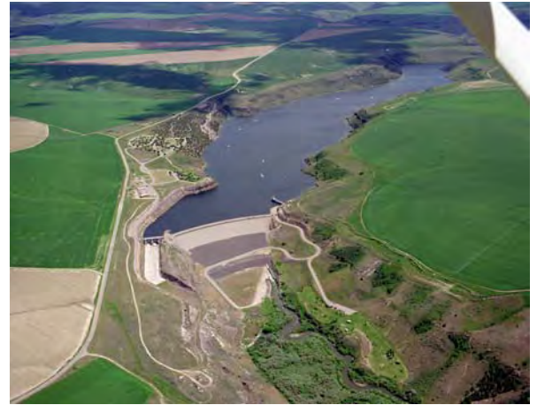
Photo 3-2. Juniper Park is located upstream of Ririe Dam; Creekside Park is located immediately downstream.
