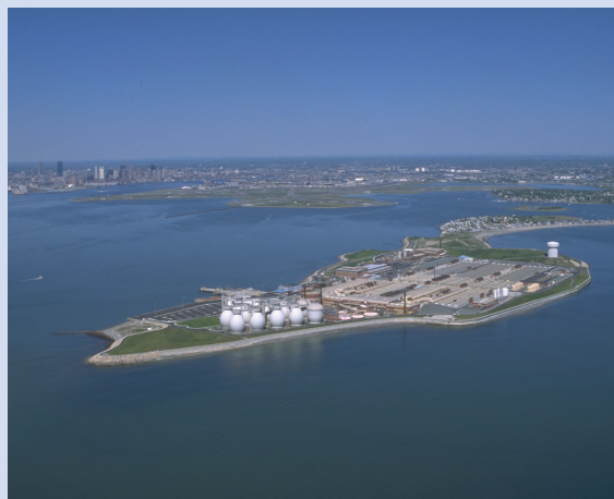
Figure: Deer Island Sewage Treatment Plant. Image courtesy of Massachusetts Water Resources Authority.
