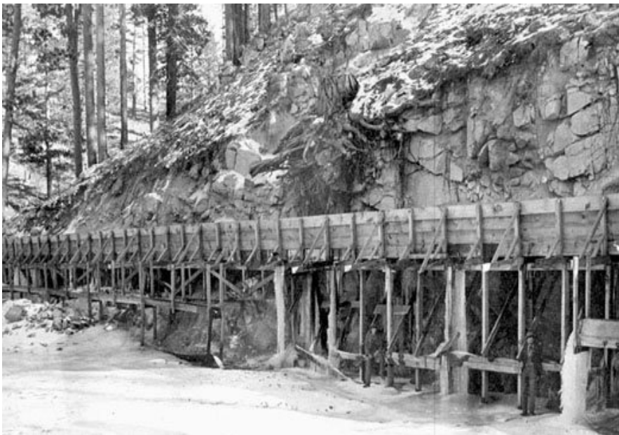
Water diversion flume, Lake Arrowhead, early 1900s (The Photoworks 2004).
