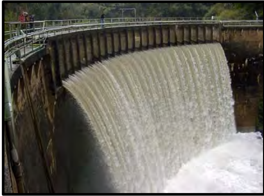
San Clemente Dam, Carmel River
