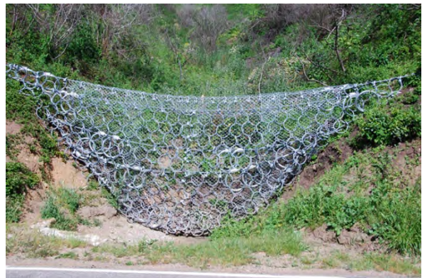
Big Sur Coast – Post-Fire Debris Control Structure (above Highway 1)
