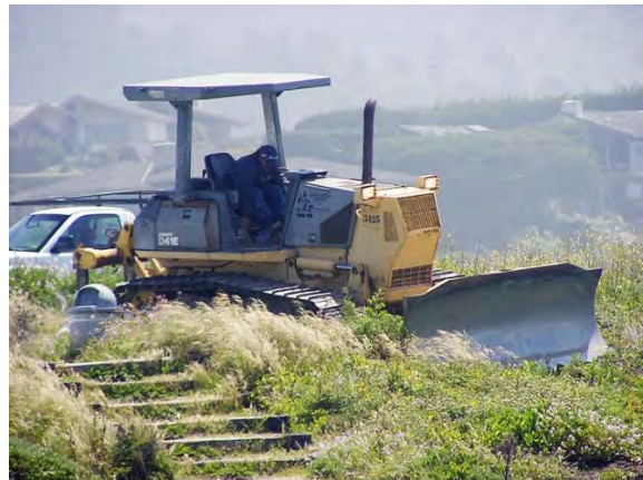
Flood Control Work –Carmel River Estuary
