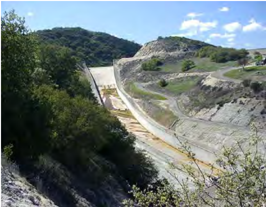
San Antonio Dam
