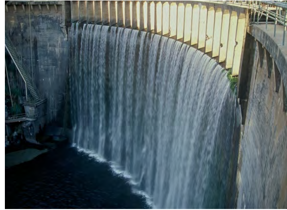
San Clemente Dam
