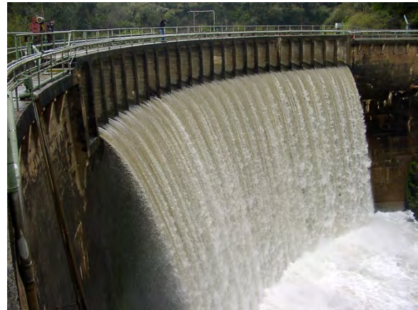
San Clemente Dam –Carmel River
