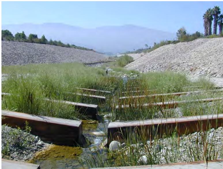
Figure 3. Santa Paula Creek Flood Control Project fish ladder on October 7, 2003 (2.8 cfs, daily average discharge) approximately one year following construction.
