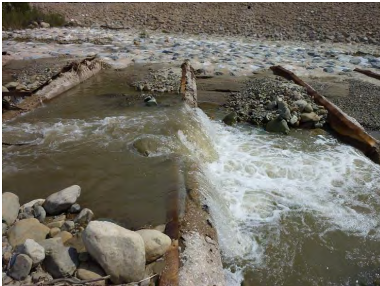
Figure 11. Santa Paula Creek Flood Control Project fish ladder on March 10, 2011.
