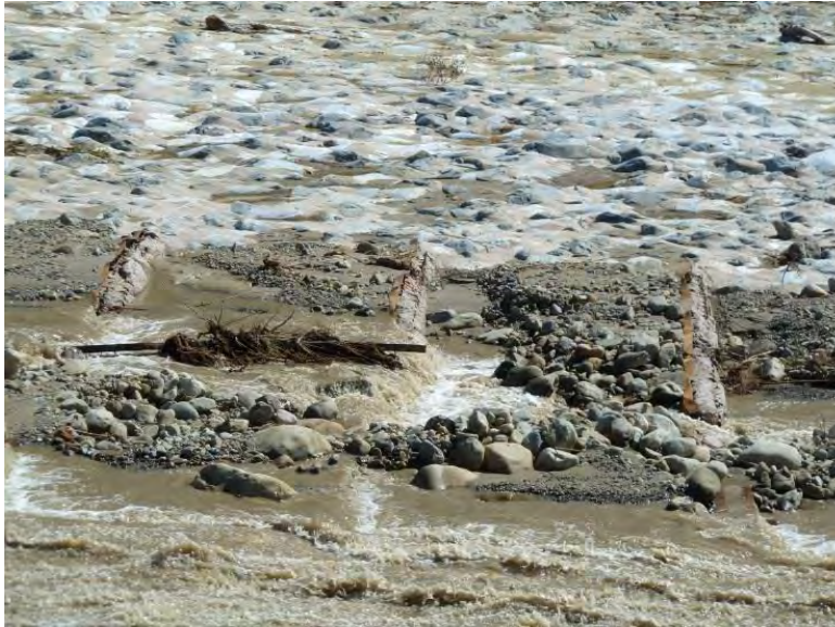
Figure 13. Santa Paula Creek Flood Control Project fish ladder, March 28, 2011 (244 cfs daily average flow) following a peak flow of 12,500 cfs on March 20, 2011.
