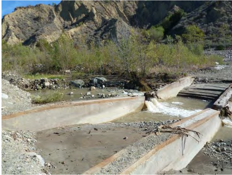
Figure 4. Santa Paula Creek Flood Control Project fish ladder on March 20, 2012 (~8 cfs) following the first stormflow event (677 cfs) of water-year 2012 on March 17, 2012.
