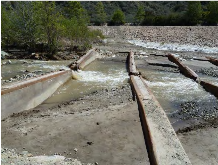
Figure 5. Santa Paula Creek Flood Control Project fish ladder on April 16, 2012 (~23 cfs) following storm flow events on March 17 (677 cfs), March 25 (190 cfs), and April 13 (793 cfs).
