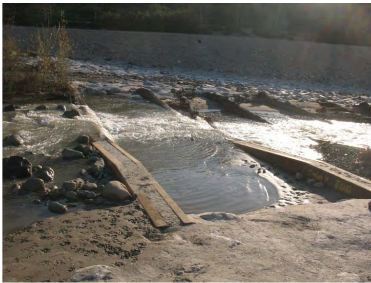
Figure 9. Santa Paula Creek Flood Control Project fish ladder, February 18, 2010 (~28 cfs).
