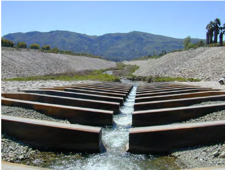
Figure 1. Santa Paula Creek Flood Control Project fish ladder, March 3, 2003 (8.9 cfs average daily discharge).
