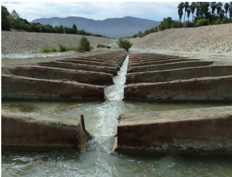
Figure 2. Santa Paula Creek Flood Control Project fish ladder, August 26, 2011 (5 cfs), approximately two months following maintenance (sediment removal) and prior to any storm flows.
