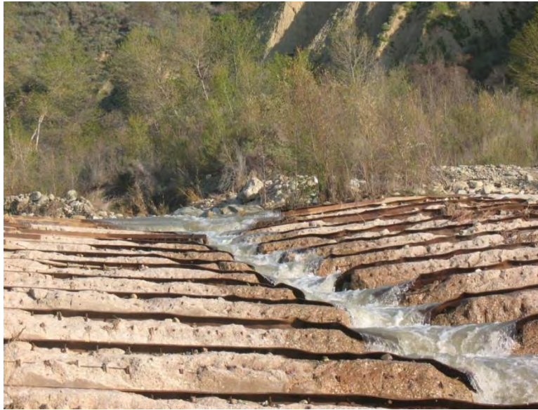
Figure 8. Santa Paula Creek Flood Control Project fish ladder, February 18, 2010 (~28 cfs).
