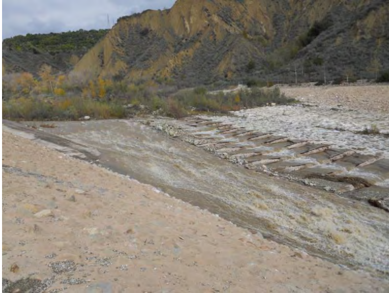
Figure 10. Santa Paula Creek Flood Control Project fish ladder, December 23, 2010 (150-175 cfs).
