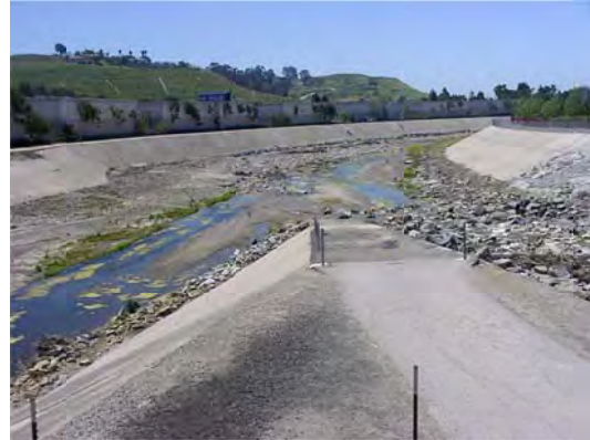
Flood Control—San Juan/Arroyo Trabuco Creeks
