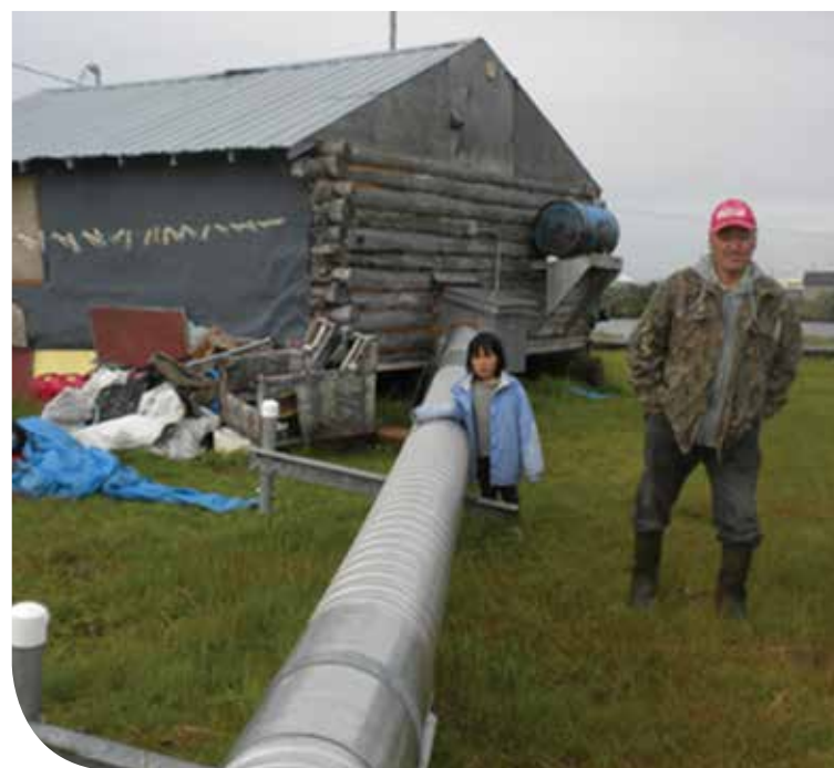
Rising temperatures are causing damage in Native villages in Alaska as sea ice declines and permafrost thaws. Resident of Selawik, Alaska, and his granddaughter survey a water line sinking into the thawing permafrost, August 2011.
