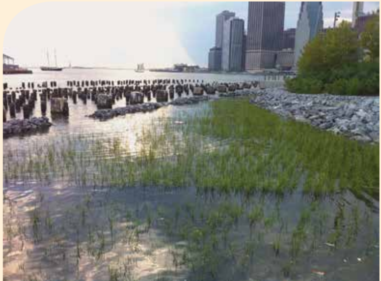
A coastal ecosystem restoration project in New York City integrates revegetation (a form of green infrastructure) with bulkheads and rip-rap (gray or built infrastructure). Investments in coastal ecosystem conservation and restoration can protect coastal waterfronts and infrastructure, while providing additional benefits, such as habitat for commercial and recreational fish, birds, and other animal and plant species, that are not offered by built infrastructure.
