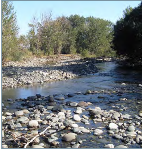
Nash Ditch, a man-made diversion before screen construction.
