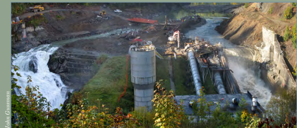
The Elwha Dam during the first phase of deconstruction.
