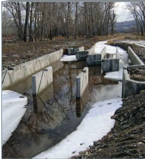
Construction of the fish screen.
