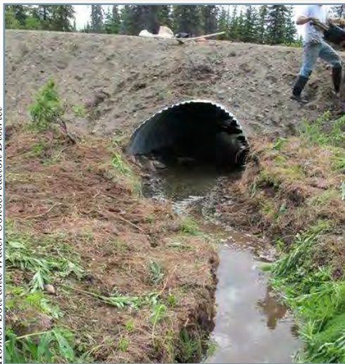
The finished culvert has a natural streambed and allows for fish passage.
