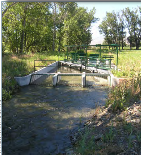
The finished diversion that prevents entrainment by fish in the irrigation canal.
