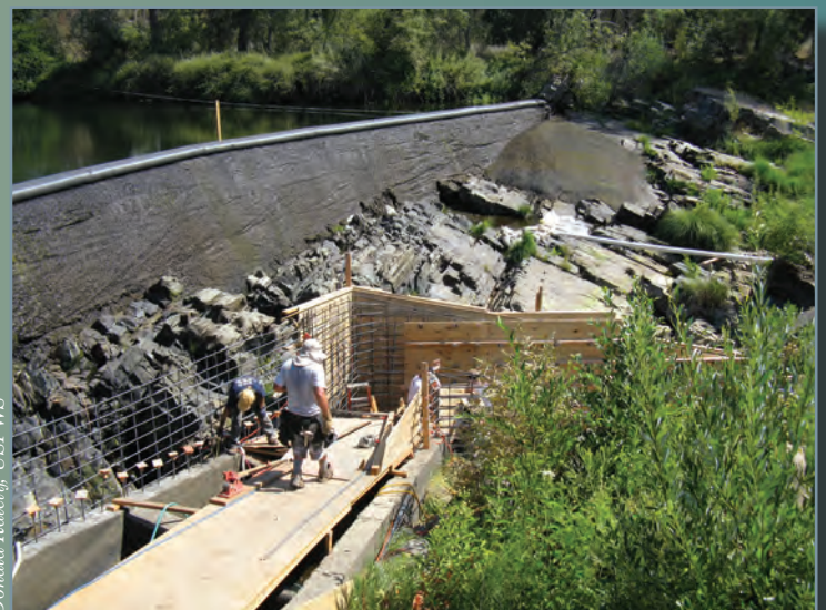
Fisheries Foundation of California constructing a fish ladder on the Cosumnes river, CA
