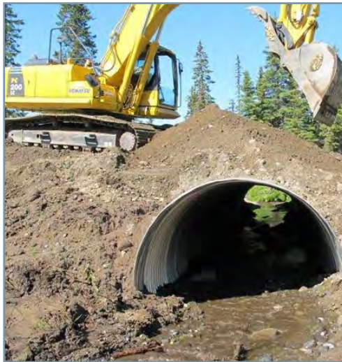
Construction of the new fish friendly culvert.
