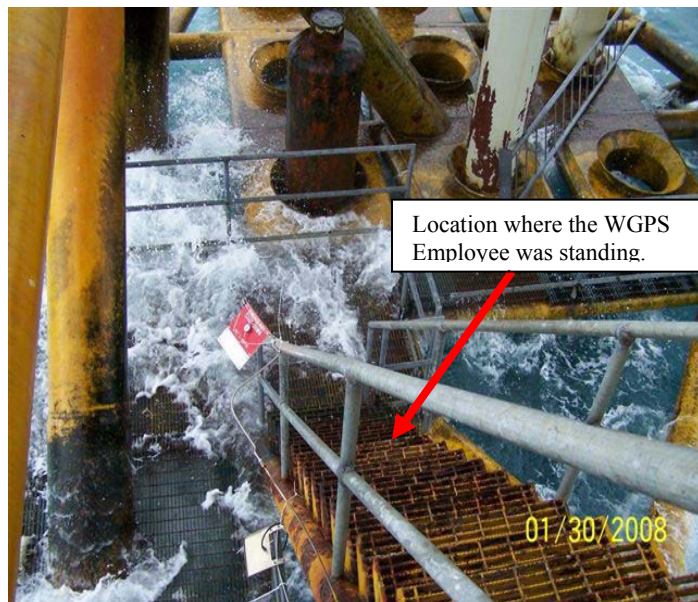
Figure 3: Photo of the WGPS Employee's location on stairs leading to boat landing.
