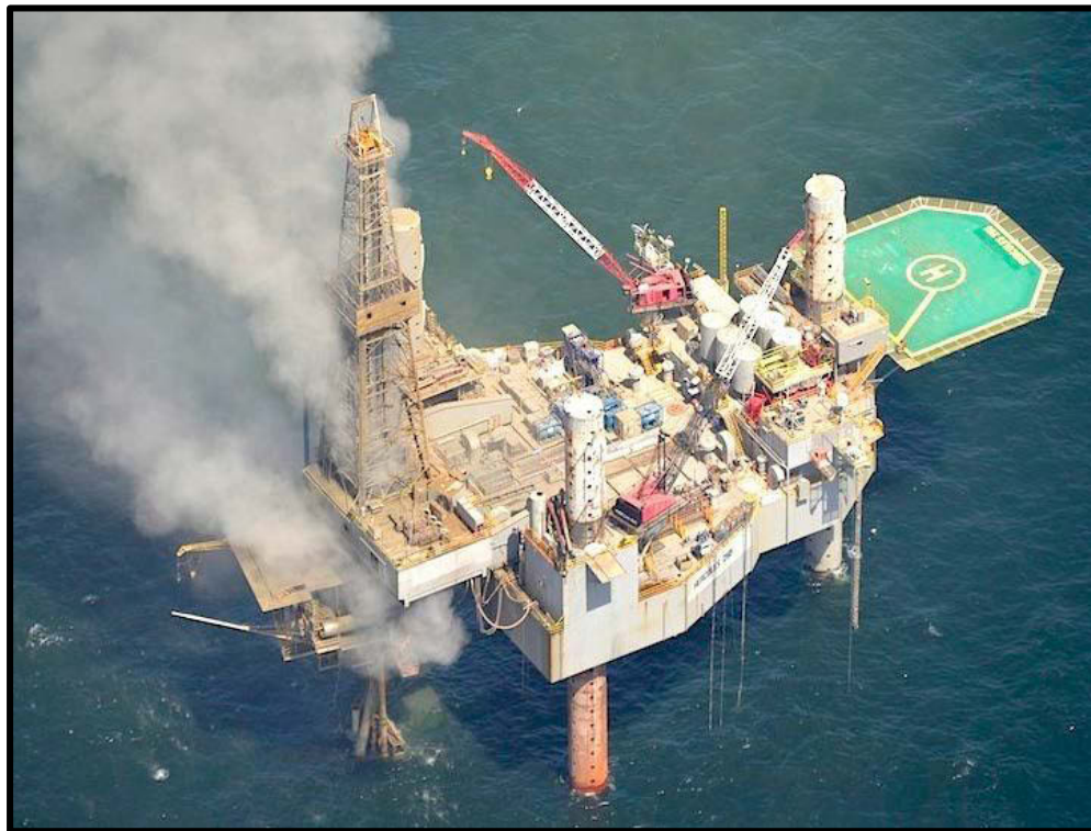
Figure 4: Hercules Rig 265 cantilevered over ST-220 “A” Platform
