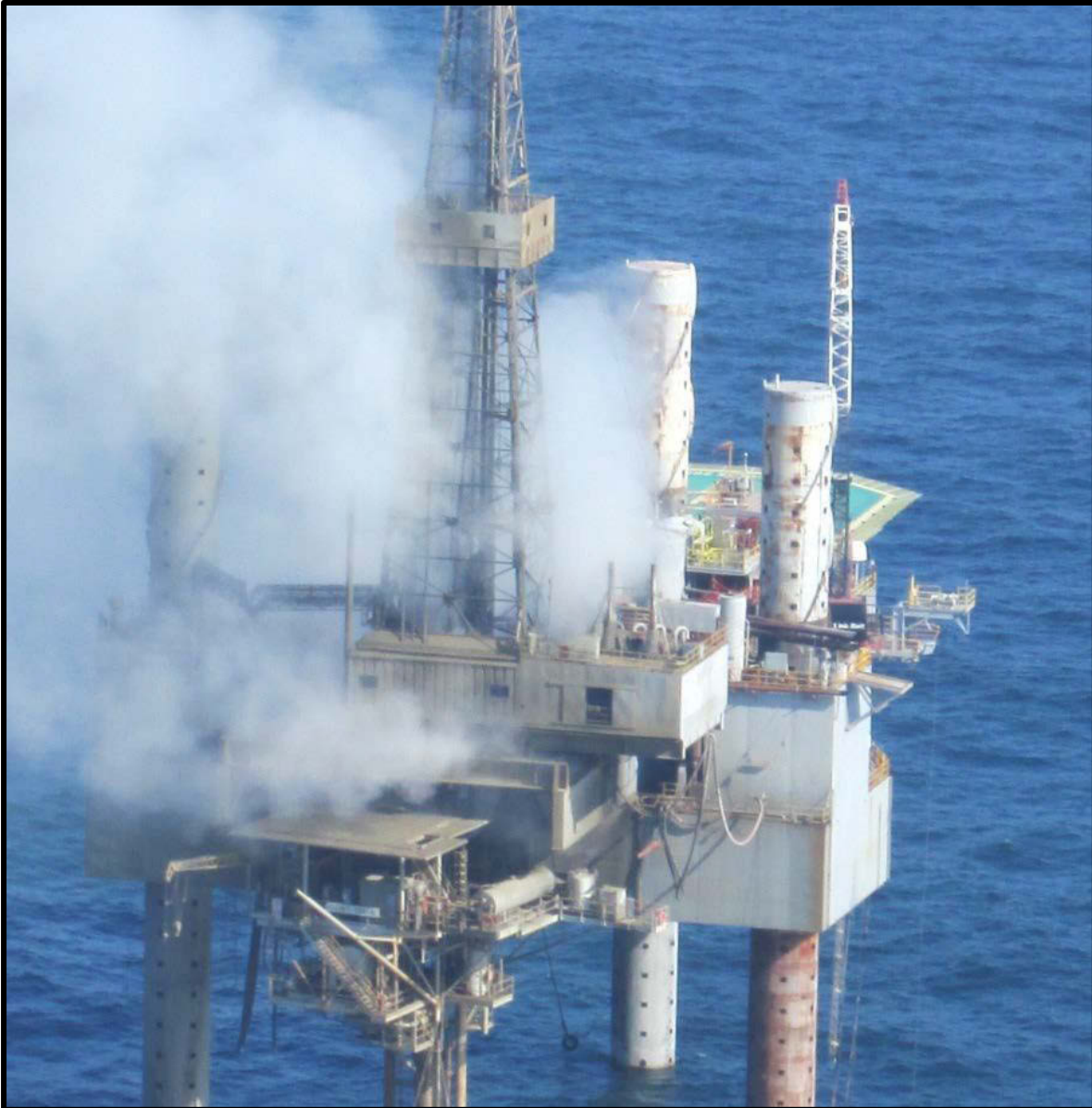
Figure 29: Rig and Platform after abandonment and loss of control
