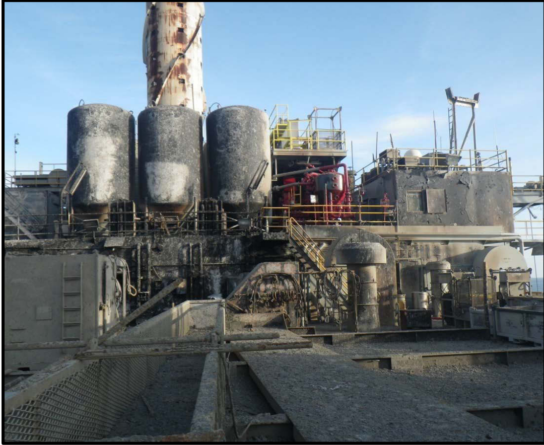
Figure 36: View of MODU looking forward, after Well bridged.
