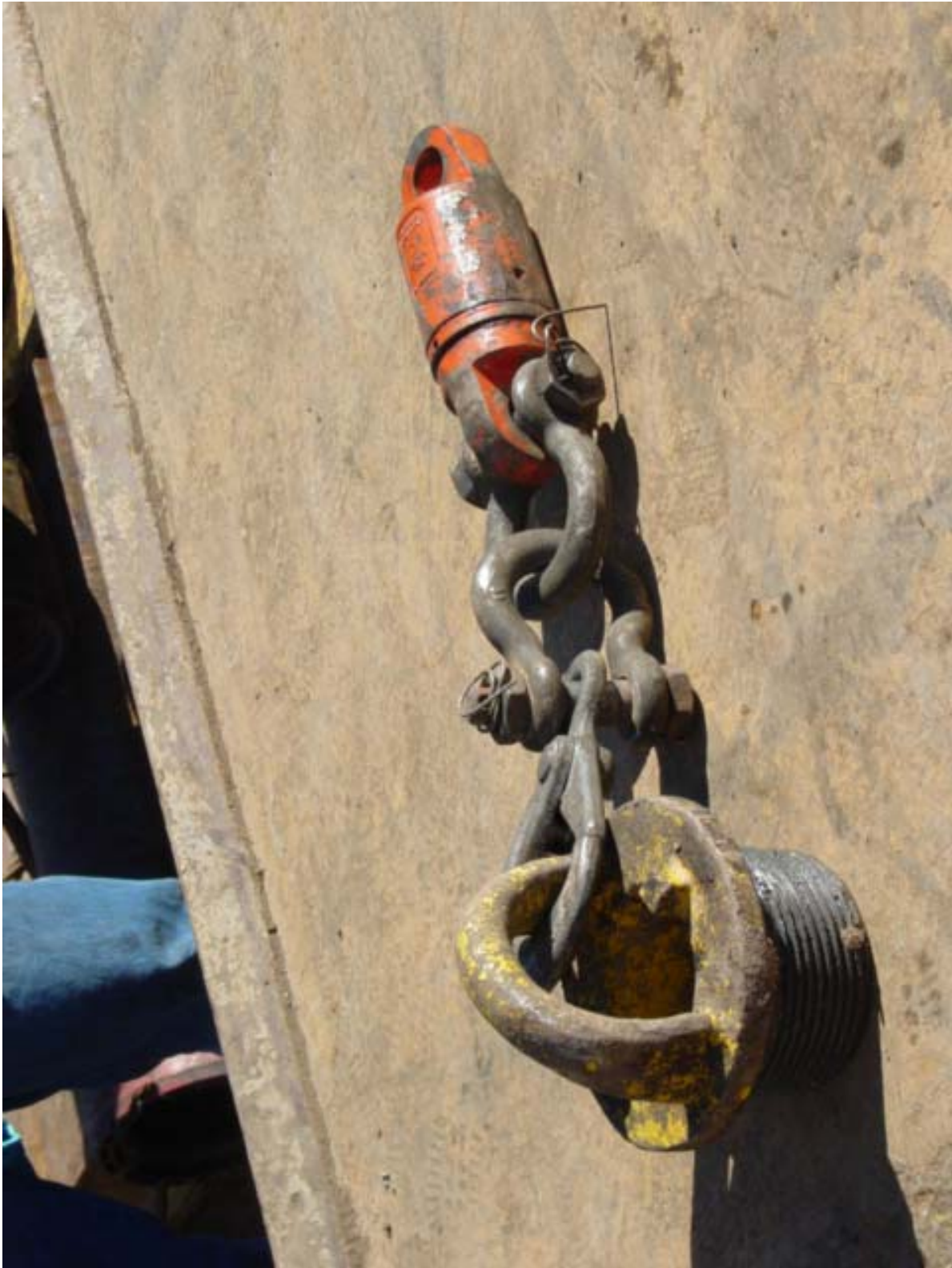
Photo of Lifting Sub that Replaced the Nylon Strap
