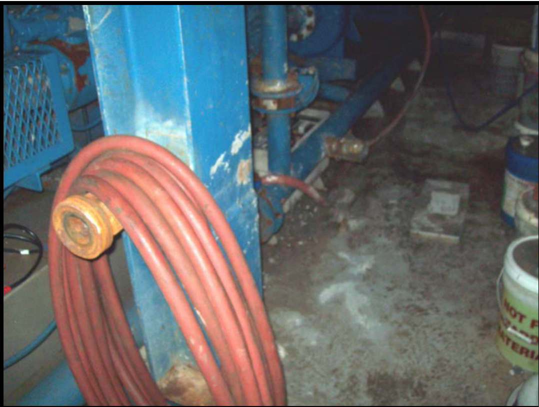
Figure 10: Deck condition immediately after Incident
