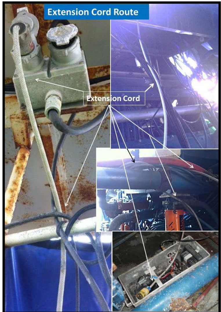
Figure 19: Extension Cord, from Outlet to Battery Box
