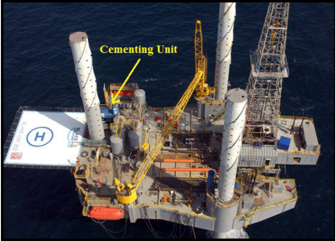
Figure 4: Rig 202 and location of Cementing Unit Skid
