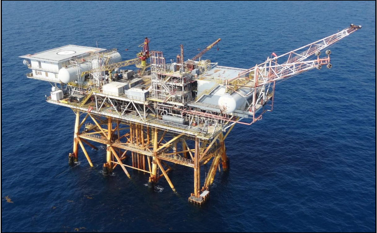
Figure 2: Pre-Incident Aerial Photo of Vermilion Block 200 Platform “A” (Photo from Talos/ERT-OFS June 28, 2012 Site Visit)
