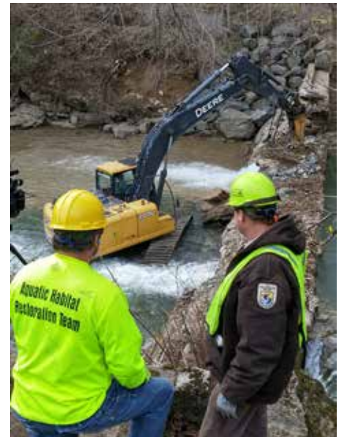
Removal of dam to improve fish passage.
