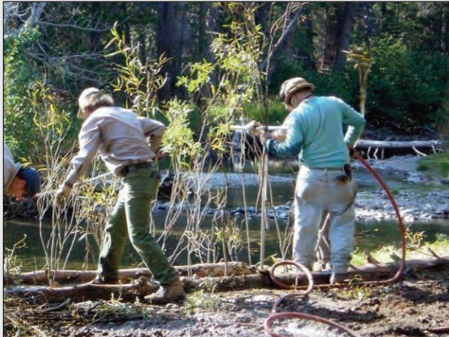
Restoring and monitoring degraded streambanks along the Middle Fork of the San Joaquin River in Devils Postpile National Monument (California).
