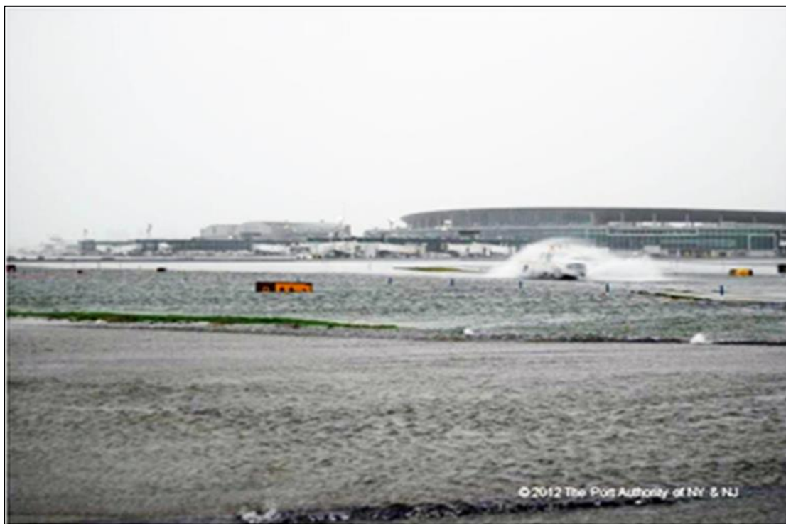
Figure 1: LaGuardia Airport during Sandy. Source: The Port Authority of New York and New Jersey
