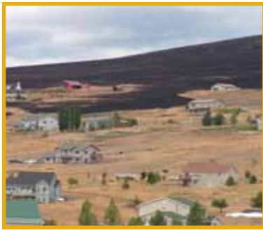
The Black Cat Fire moved out of the timber down a dry, grassy slope into the wildland-urban interface a few miles northwest of Missoula, MT; August 2007. Photo taken by Mark D. Roper, San Juan National Forest, CO.
