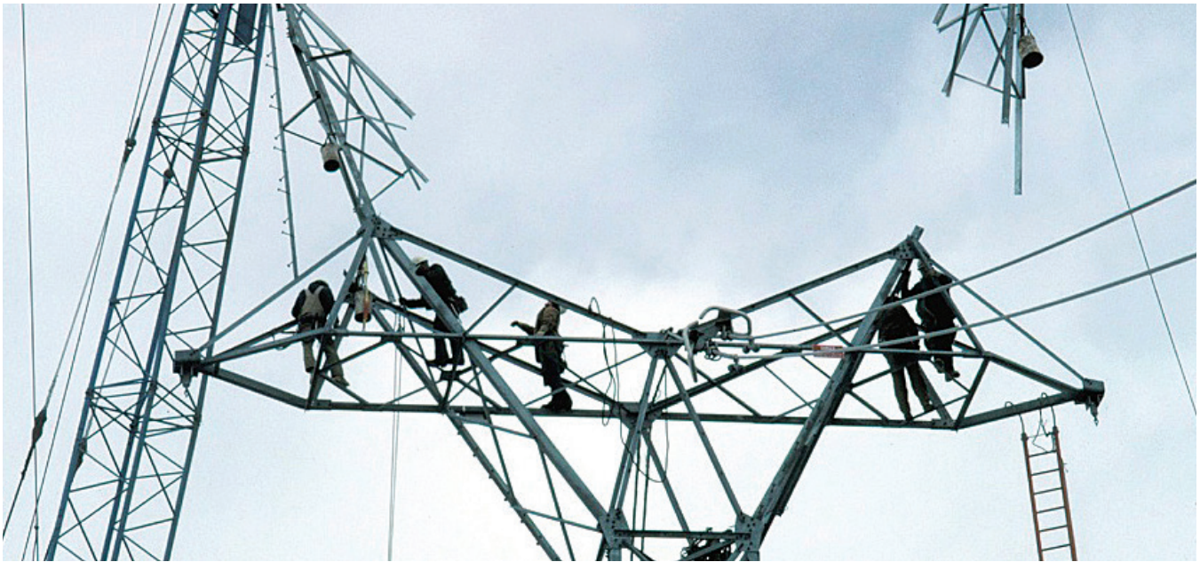
A crew bolts together a new 500-kilovolt transmission tower.
