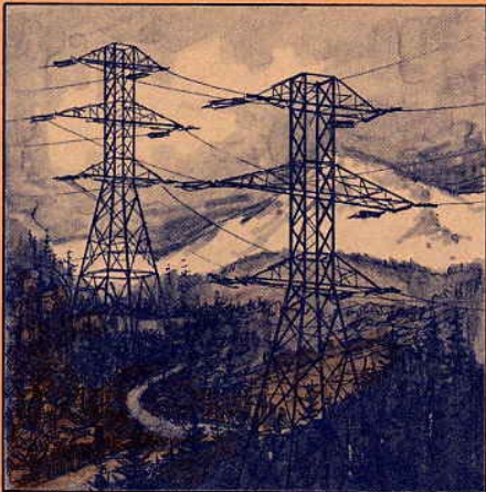
Steel tower transmission line.
