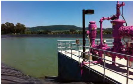
Construction (above) and the completed (below) 100 acre-foot capacity recycled water reservoir by the Sonoma Valley County Sanitation District, part of a Title XVI project to reduce reliance on groundwater supplies. Photos courtesy of North Bay Water Reuse Authority, all rights reserved, 2016.
