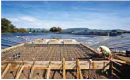
Construction (above) and the completed (below) 100 acre-foot capacity recycled water reservoir by the Sonoma Valley County Sanitation District, part of a Title XVI project to reduce reliance on groundwater supplies. Photos courtesy of North Bay Water Reuse Authority, all rights reserved, 2016.
