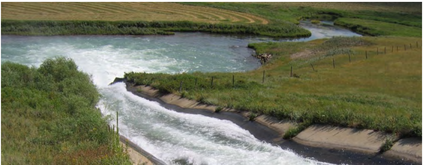
Drop chute in the St. Mary River Basin. Reclamation photo.
