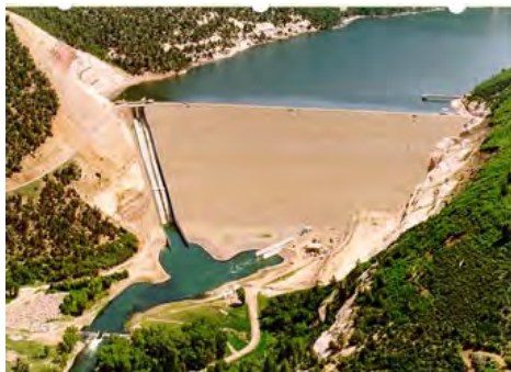
McPhee Dam is located on the Dolores River a tributary of the Colorado River. Reclamation photo.
