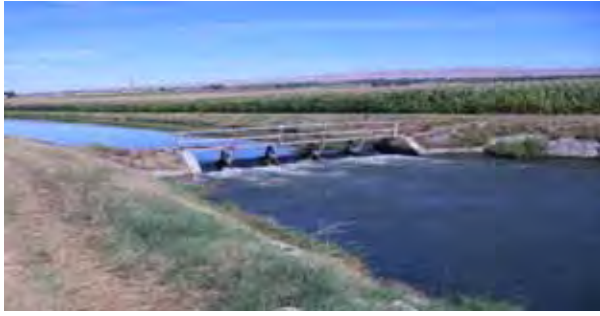
Figure 1. Picture of a manual check structure used to control water elevation are dangerous to adjust and laborintensive.
