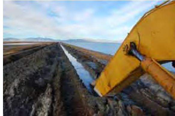
Figure 2 - Contractor completes the cutoff wall through the dam crest – November 21, 2008
