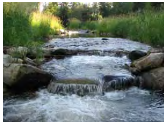
Figure 2. The old push-up diversion dam was replaced with a series of three boulder weirs that allow upstream passage for adult and juvenile fish.
