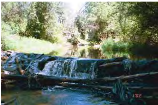
Figure 1. Before it was removed, the Thurlow transfer ditch push-up diversion dam blocked fish passage to upstream spawning and rearing areas.
