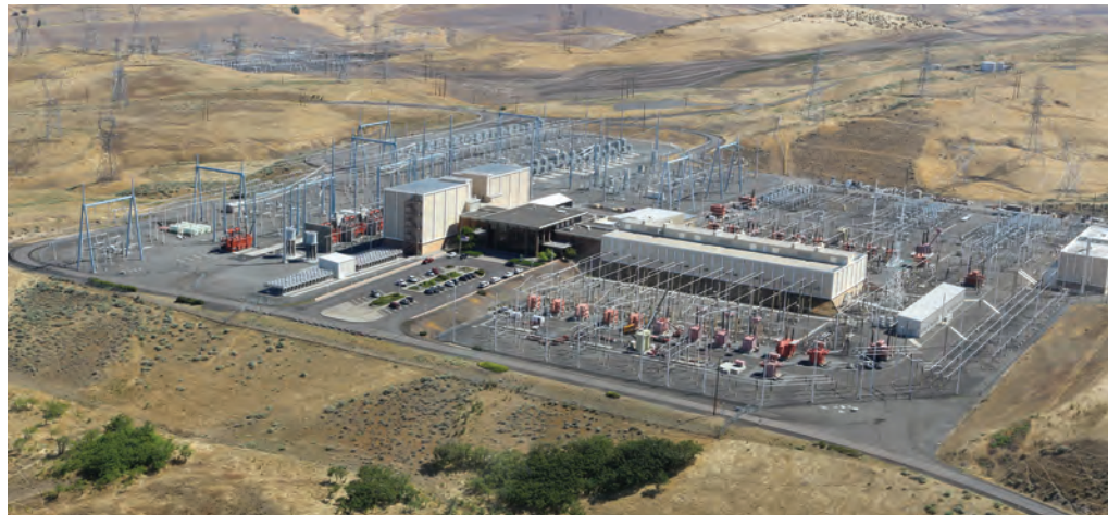
Celilo Converter Station after modernization.
