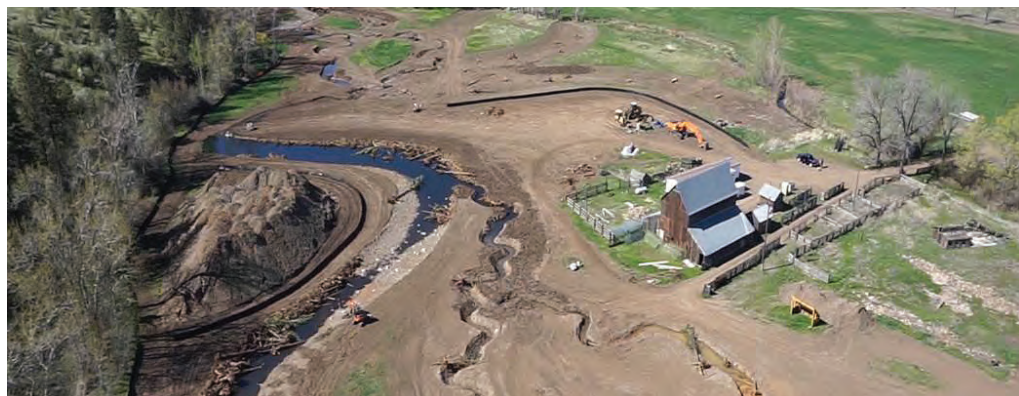
The Catherine Creek restoration project reconnected the creek with its floodplain, improving conditions for fish at all life stages.
