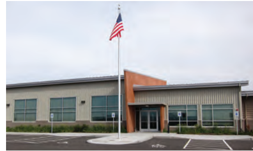
Nekitpe Maintenance Headquarters
