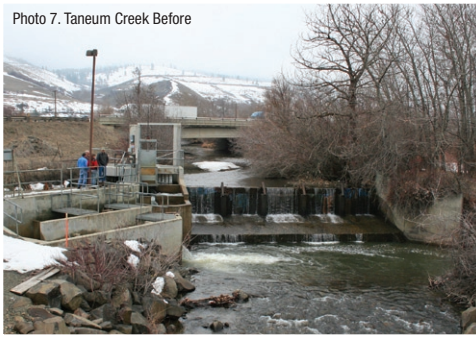
Photo 7. Taneum Creek Before
