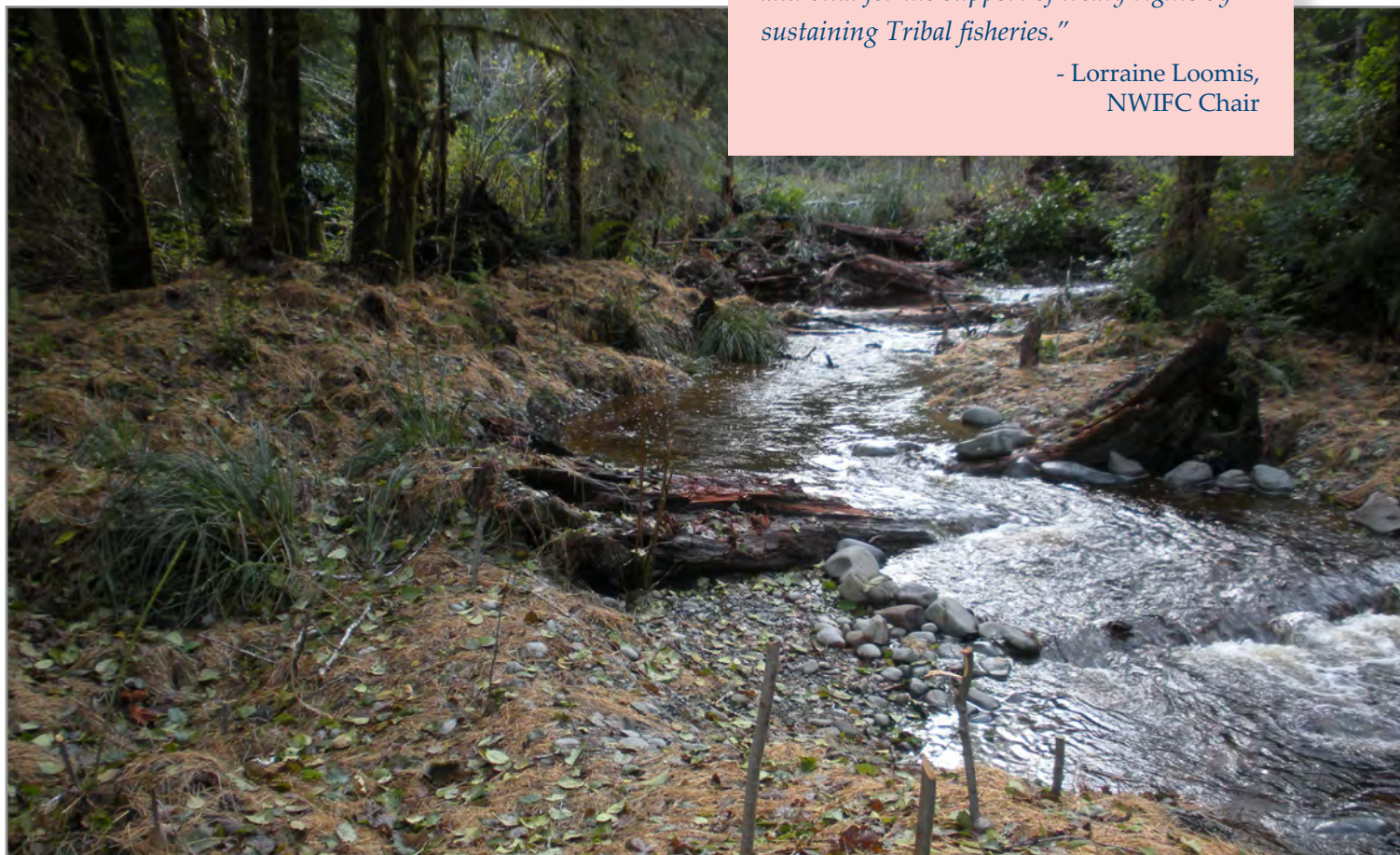
Chalaat Creek's constructed channel leads to the pond. Photo: Northwest Indian Fisheries Commission
