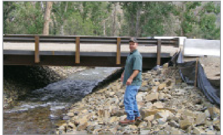
Iron Creek after culvert replacement
