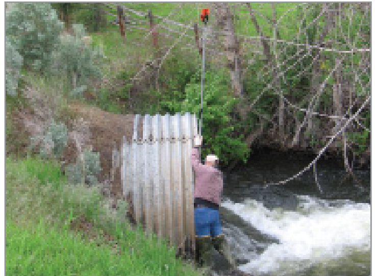
Iron Creek before culvert replacement
