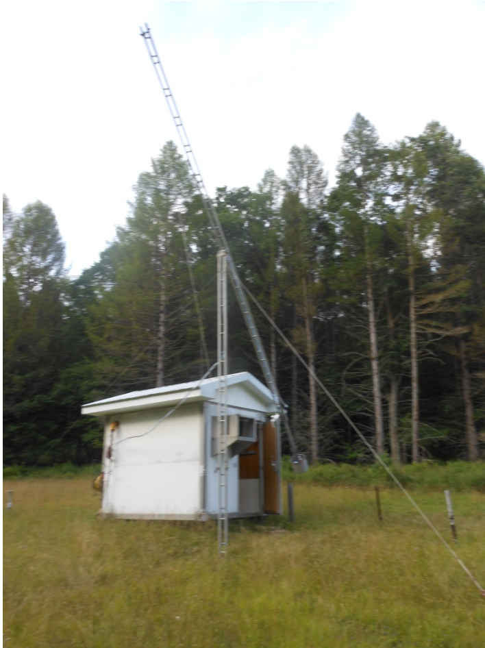
Figure 24. Lowered Flow Tower
