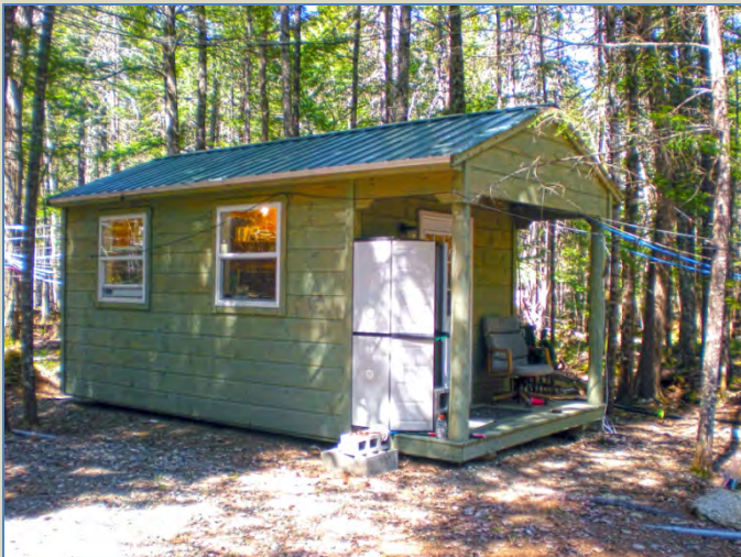
HOW191 site shelter
