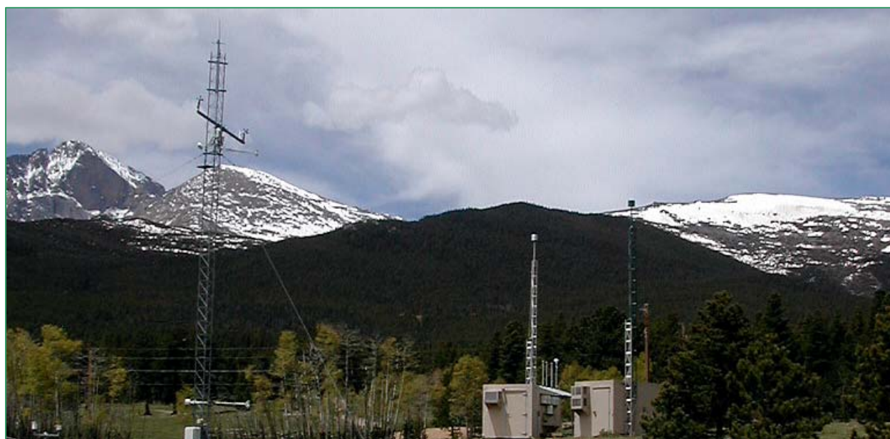
Rocky Mountain National Park, CO (ROM406/206)
