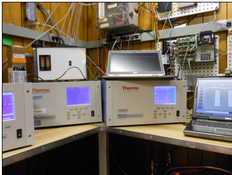
Figure 8. Analyzers inside the BFT142 Shelter
