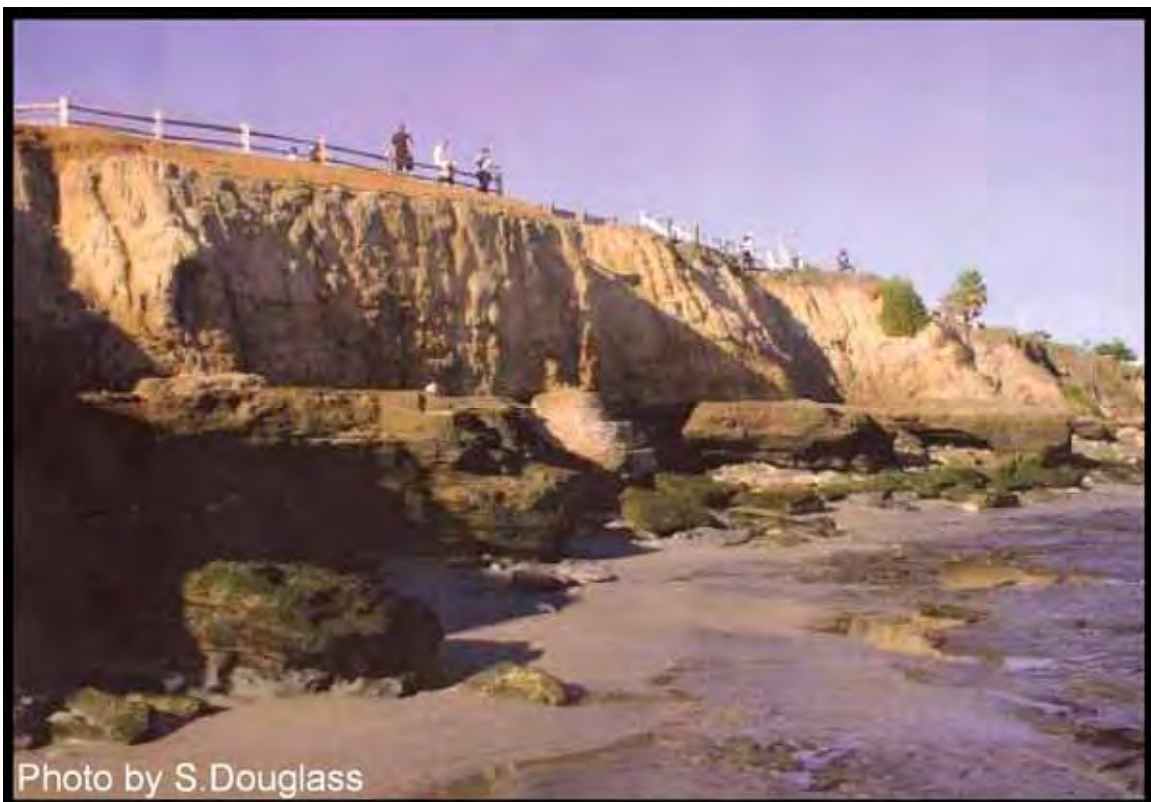
Figure 6.12. Concrete seawall designed to look like the natural rock formation built on an eroding sea cliff to protect a local road. East Cliff Drive, Santa Cruz, California
