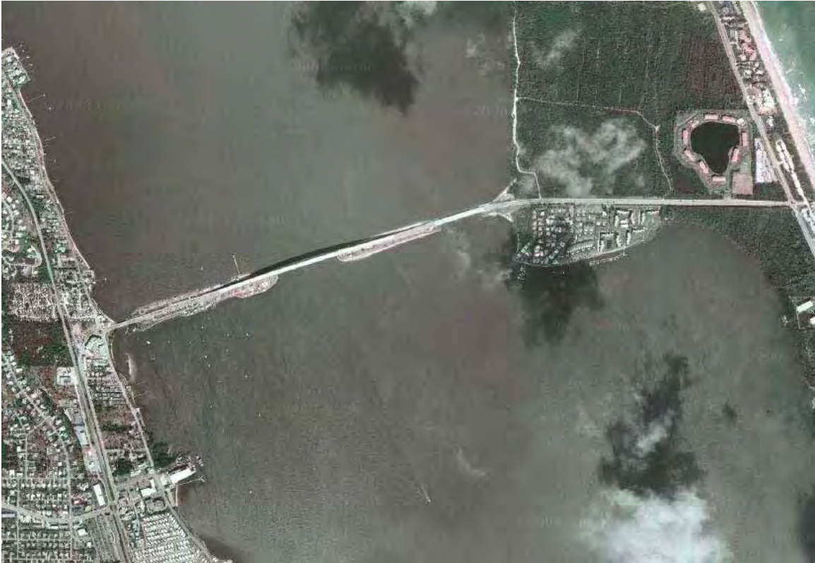
Figure 9.10. Jensen Beach Causeway bridge.
