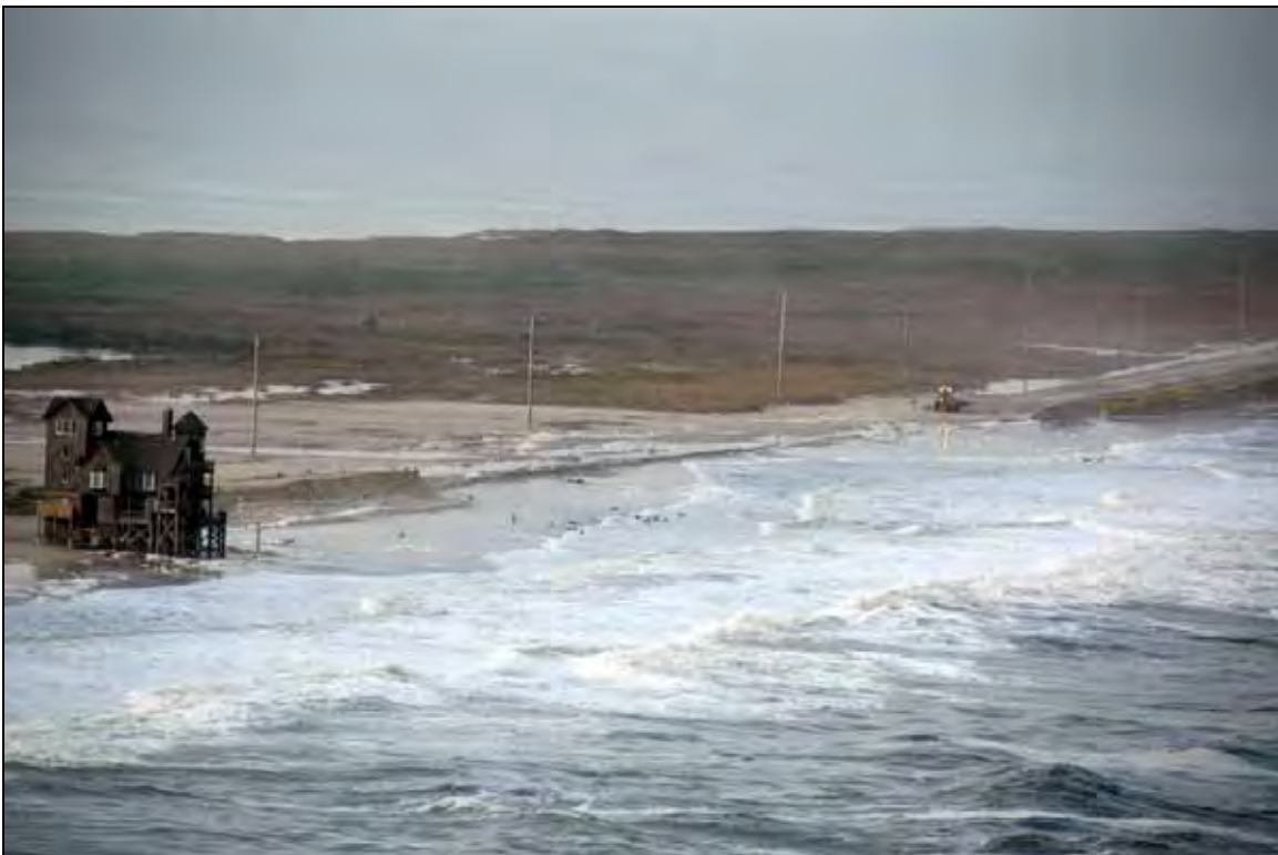
Figure 8.1. A coastal road being overwashed during a storm. North Carolina Highway 12, November 23, 2006 (North Carolina DOT photo)
