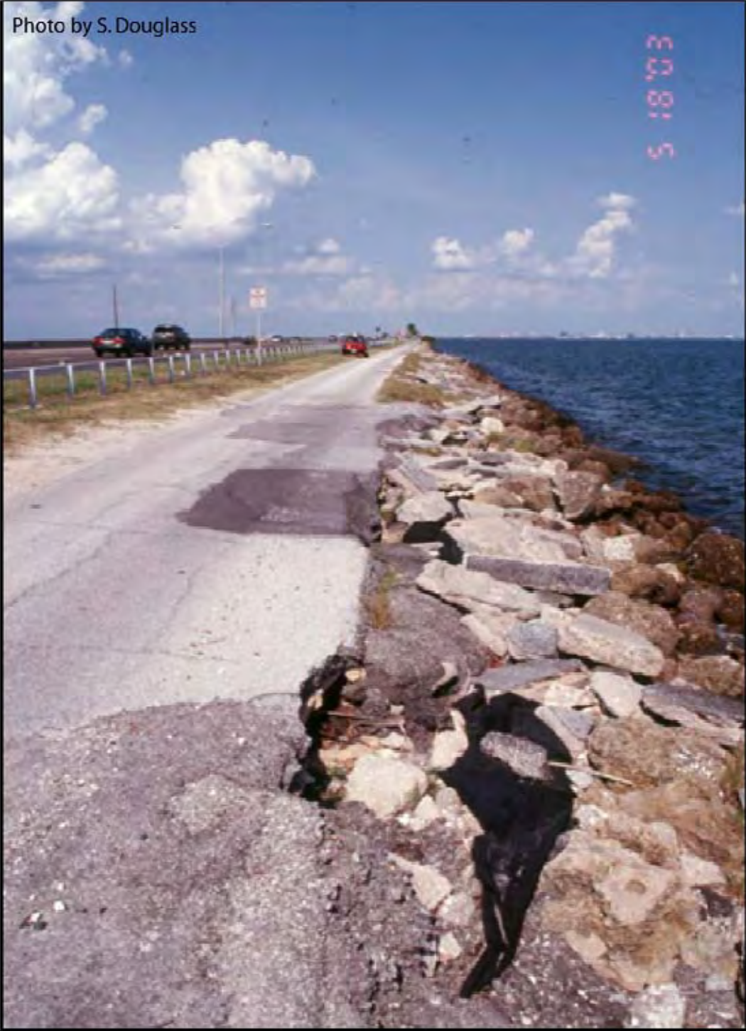
Figure 6.9. Revetment protecting a highway along a bay shoreline. Florida Highway 60, Tampa Bay, Florida (2003)
