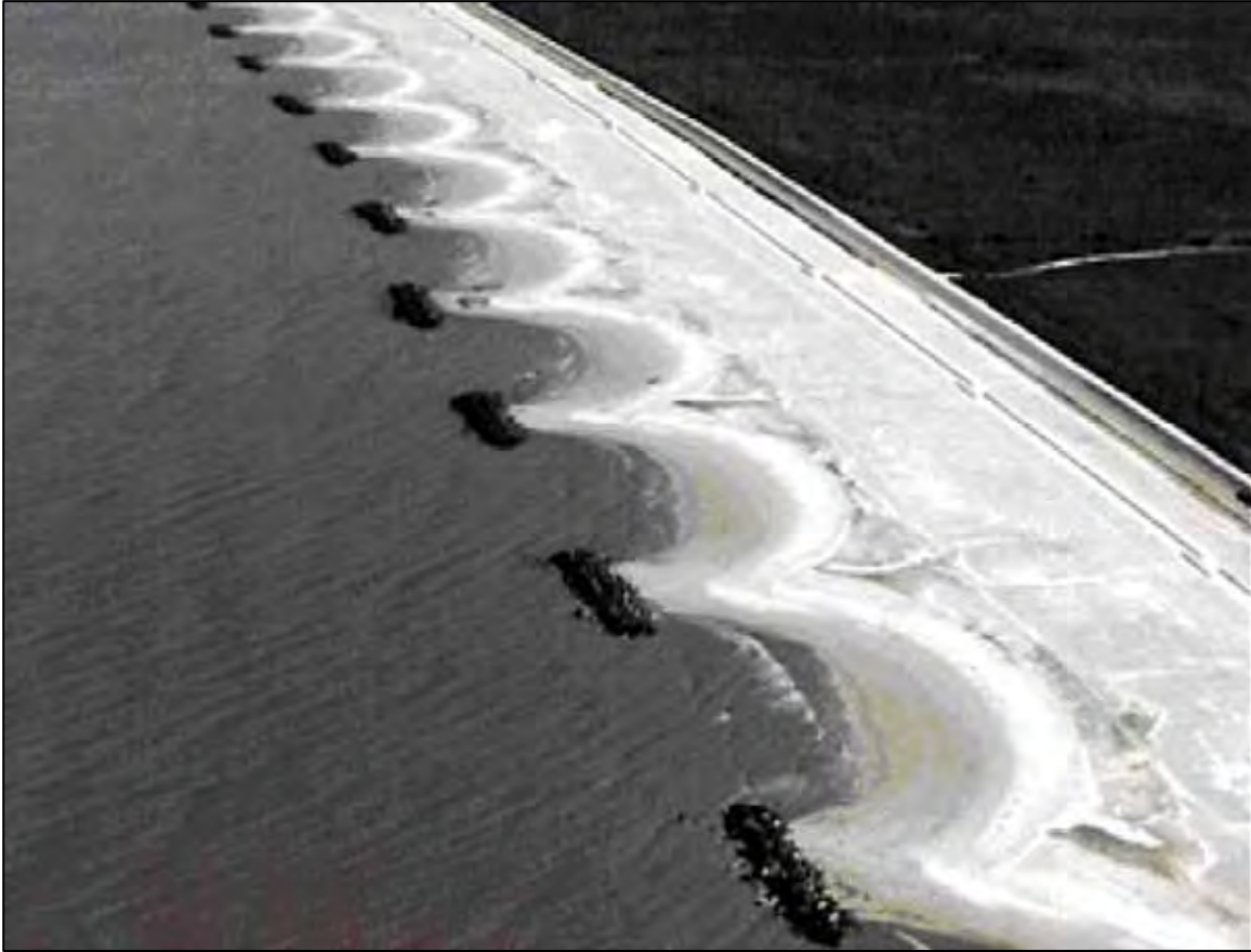
Figure 7.18. Offshore segmented breakwaters with tombolos in beach nourishment protecting a highway (Louisiana Highway 82, Holly Beach) (American Shore and Beach Preservation Association photo, circa 2003).
