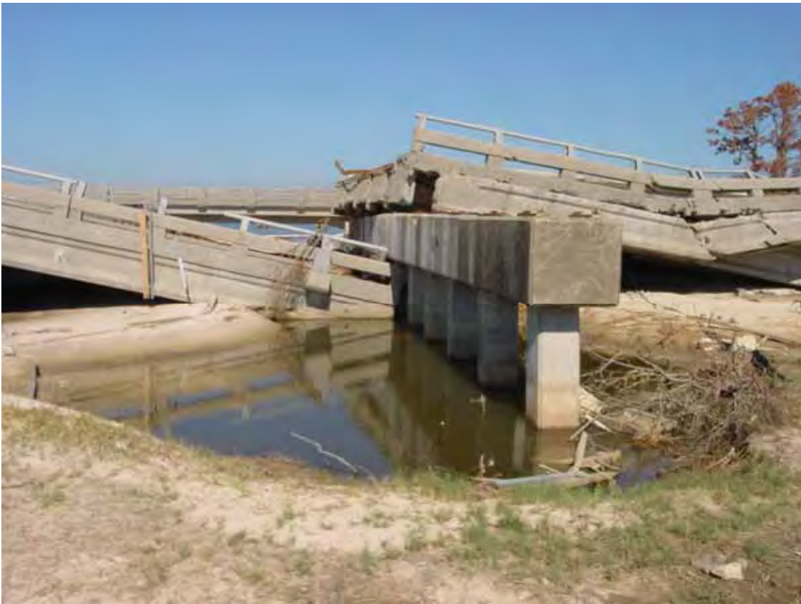
Figure 9.7. Wave scour hole formed by Hurricane Katrina.
