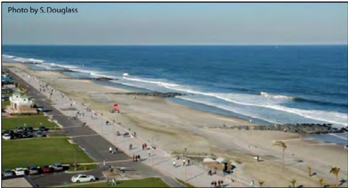
Figure 7.13. Groin field in Long Branch, New Jersey (2006)
