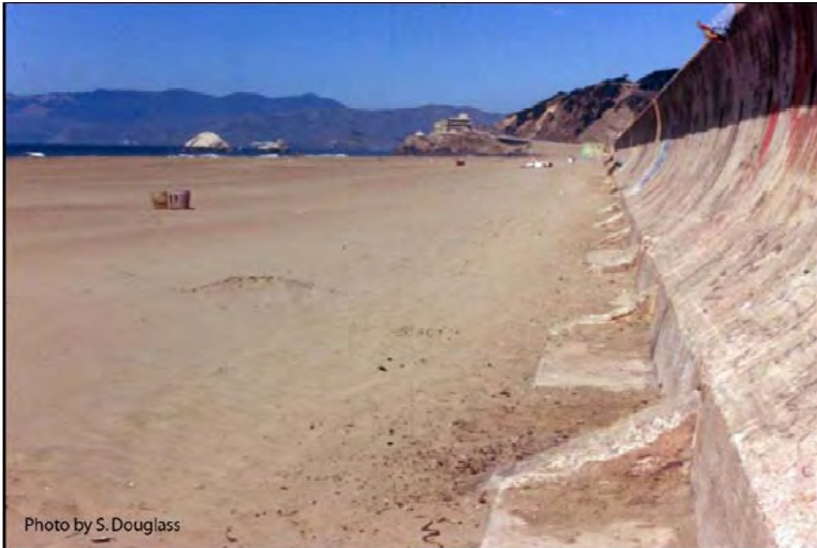
Figure 6.4. San Francisco's Great Highway Seawall. California Highway 35 (1991)
