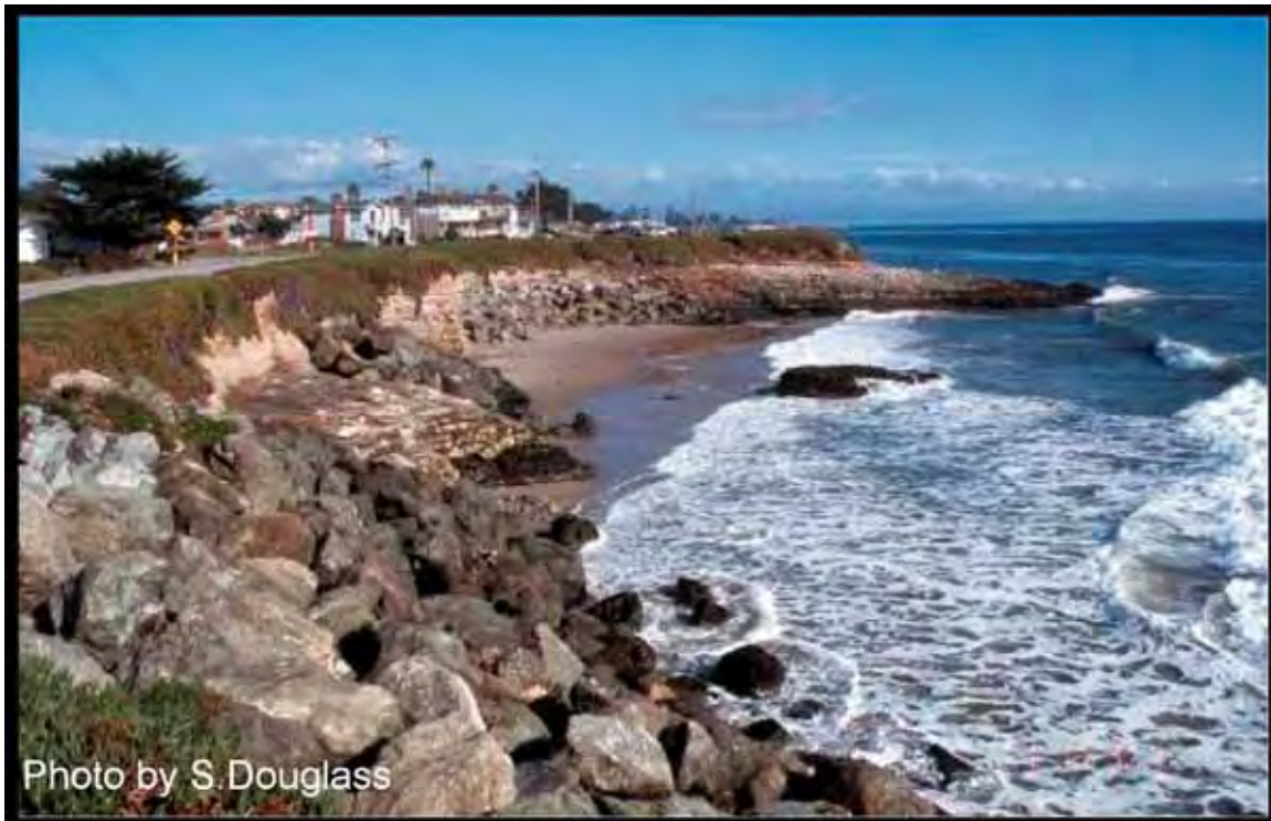
Figure 6.11. Seawall protecting a local road. West Cliff Drive, Santa Cruz, California
