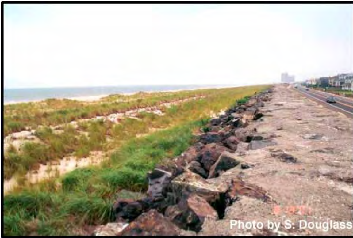
Figure 7.17. Beach nourishment seaward of a seawall protecting a road. New Jersey State Highway 35, Sea Bright, New Jersey (2001)
