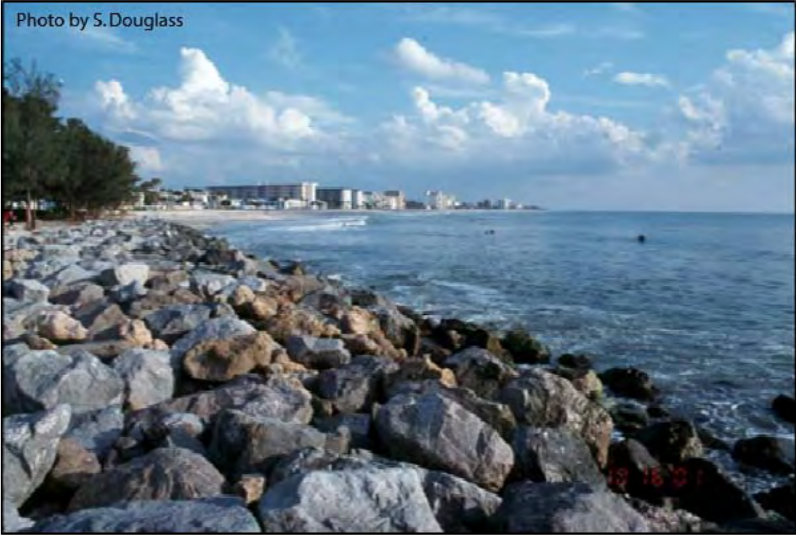
Figure 6.5. Seawall protecting a coastal highway. Venice, Florida (2001)
