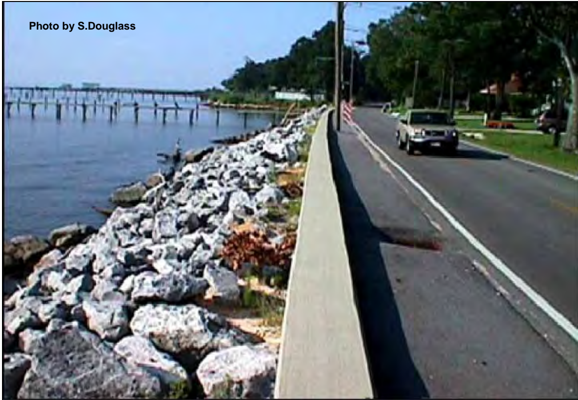
Figure 6.1. A revetment protecting a coastal highway. Bayfront Road, Mobile, Alabama (2001)
