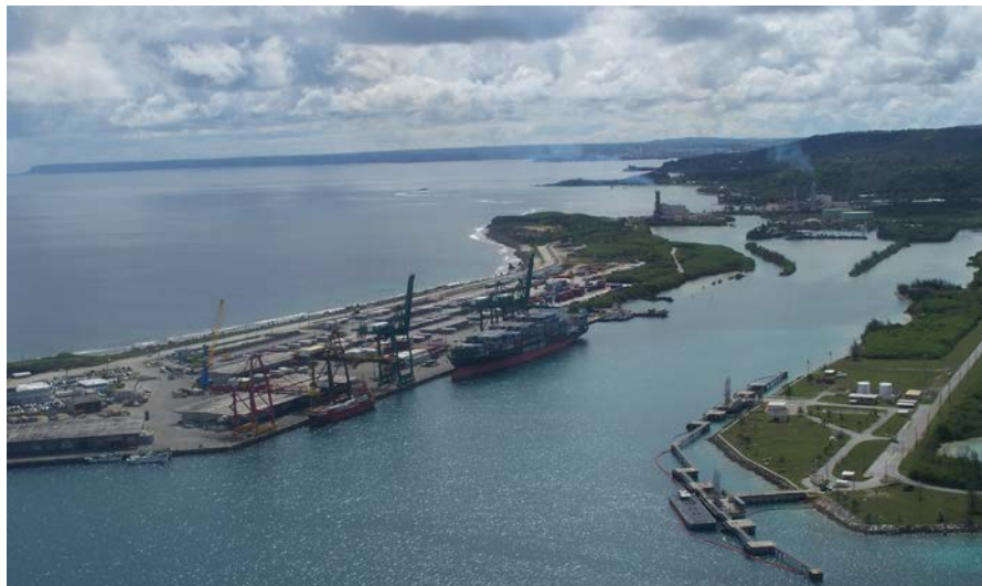
View of the commercial port area of Guam within Apra Harbor. Power plants are located at the head of the port area.
