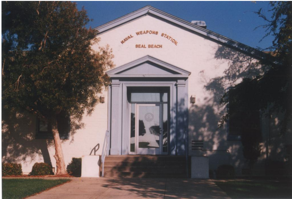
Photo 3-17. Example of architecture on Naval Weapons Station Seal Beach.
