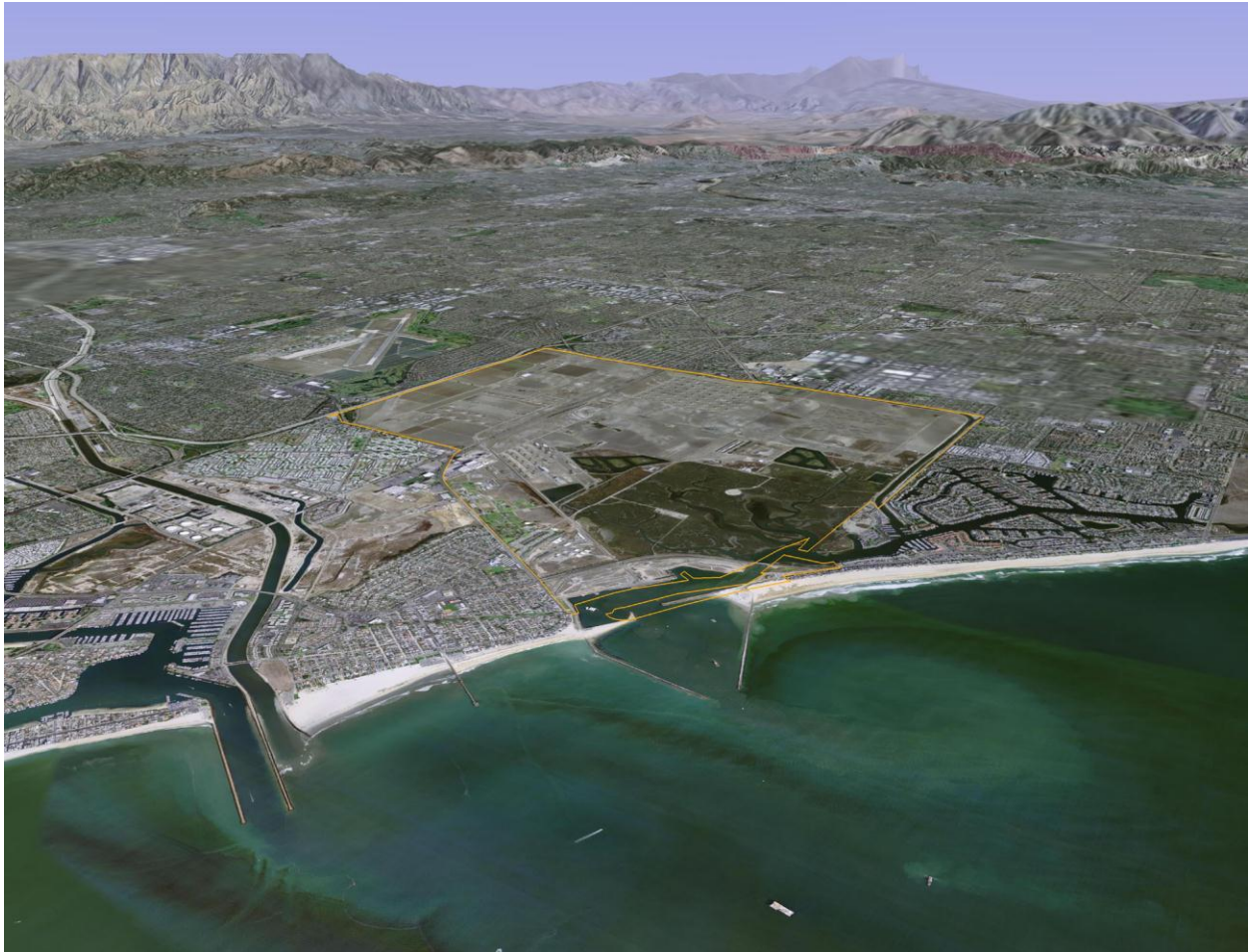
Figure 3-4. Depiction of the nearby watershed affecting Naval Weapons Station Seal Beach. Elevations are exaggerated by 100 percent. (Source: Google Image).
