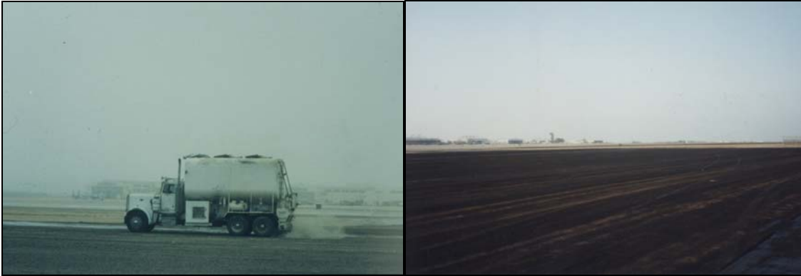
Figure 15. In 1999, the Public Works Department soil cemented 52 acres at the approach end of runways 11 and 18 to reduce the incident of runway crossings by all species of birds in this area of the airfield. (Photo by John Cummings, U.S. Department of Agriculture, National Wildlife Research Center, Fort Collins, CO, July 1999).
