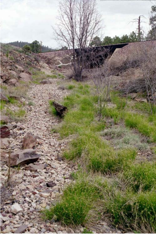
Photo 1. Site 1, drainage under railroad track.
