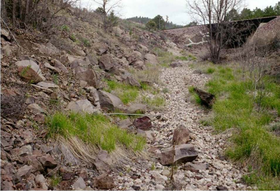
Photo 8. Area 1, drainage under railroad track.
