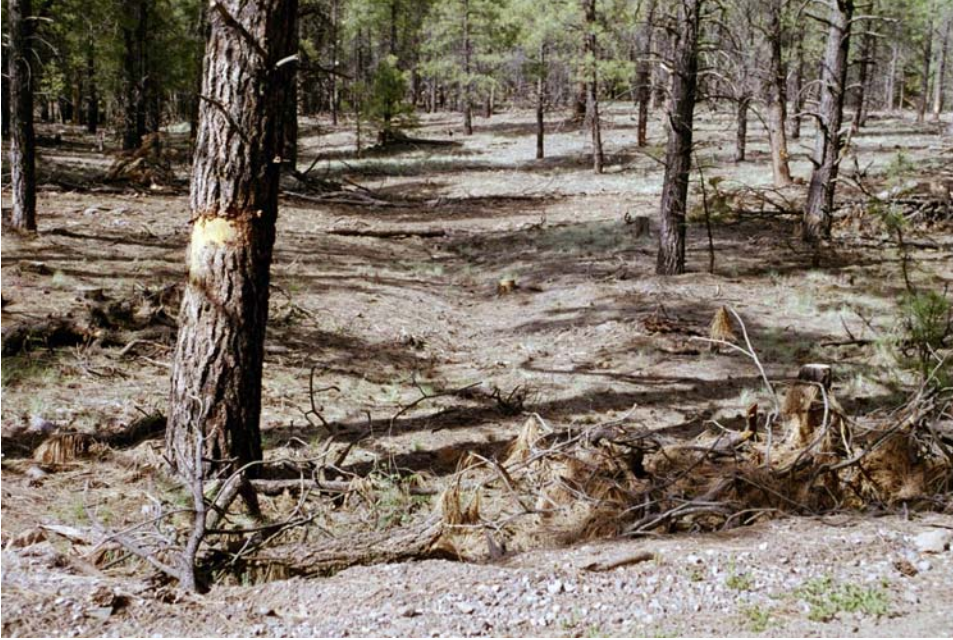
Photo 28. Area 7, Waters of U.S. Check 4, culvert downslope, eroded channel and debris.
