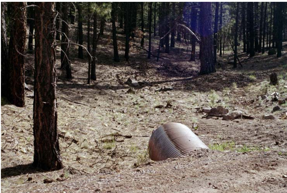
Photo 27. Area 8, culvert upslope, Waters of U.S. Check No. 4, no deposition, no defined bed and bank.
