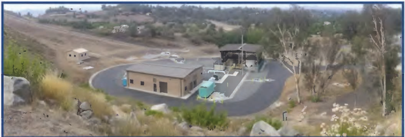
Red Mountain Reservoir Ultraviolet Treatment (UV) Plant
