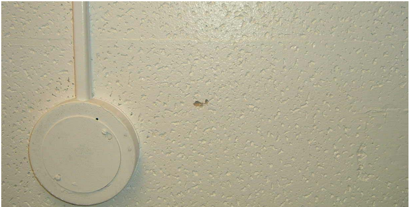
Older ceiling panels (above) and acoustic materials may contain asbestos.
