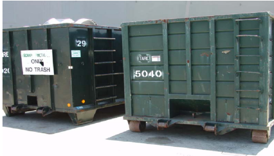
Figure 21.4 shows the staging of the roll-offs on the pier during CBR filter replacement. Note, the roll-off containing the Category Two, (recyclable aluminum) filters are identified as scrap metal.
