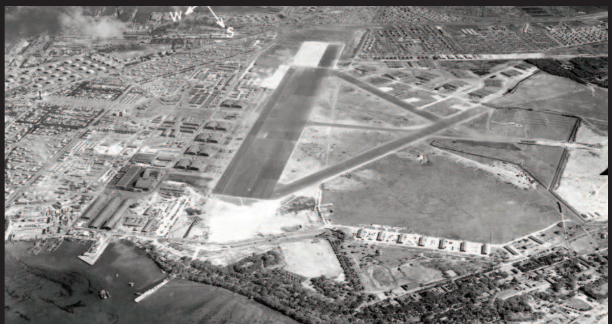
Photo courtesy of Hawaii Department of Transportation, Airports Division Former Hickam Field is shown here in an aerial photo dated Nov. 16, 1943 (72 years ago this month).
