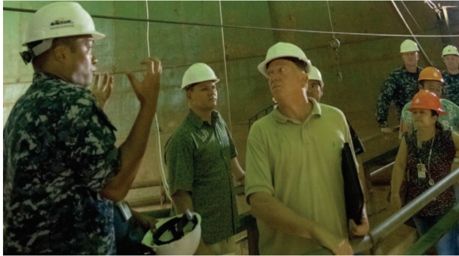
U.S. Navy photos by MC2 Laurie Dexter Capt. Ken Epps, left, commanding officer of NAVSUP Fleet Logistics Center Pearl Harbo briefs to Board of Water Supply representatives, Sept. 15, on a scaffold inside an empty tank.
