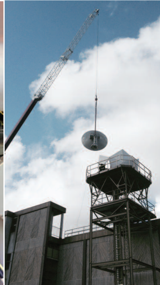
(Above) NCTAMS PAC Makalapa Tech Control personnel, Information Systems Technician 1st Class (IDW/SW) Joseph Seeley and Electronics Technician 1st Class (IDW/SW) Cameron Otejen, run initial tests on the newly installed AN/FSC-138 Navy multi-band terminal. (Above right) NCTAMS PAC Makalapa Tech Control installs the new Navy multi-band at U.S. Pacific Fleet.
