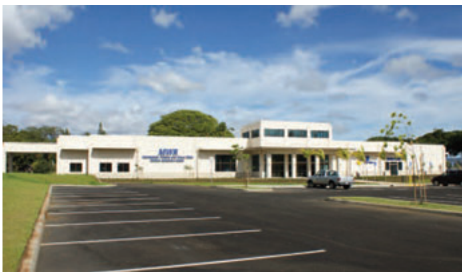
A full front view of the newly completed Navy Exchange Fleet Store at Joint Base Pearl Harbor-Hickam. U.S. Navy photo by Denise Emsley
