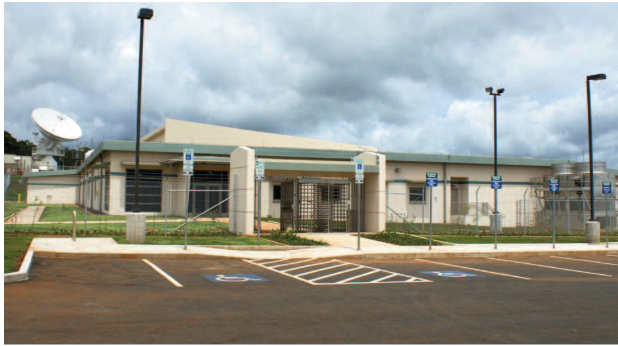
This is a front view of the U.S. Army 53rd Signal Battalion's new 28,244 square-foot wideband satellite communication operations center (WSOC) facility at Joint Base Pearl Harbor-Hickam, Wahiawa Annex, Hawaii.
