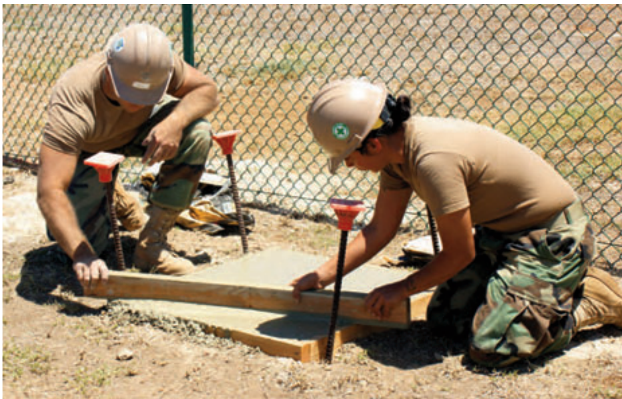
U.S. Navy photo by Thomas Obungen (Left to right) Utilitiesman 3rd Class Rodrigo Diaz and Steelworker 2nd Class (SCW) Jessica Majoy create a square concrete slab for installation of a bag dispenser at the new Ford Island Dog Park.
