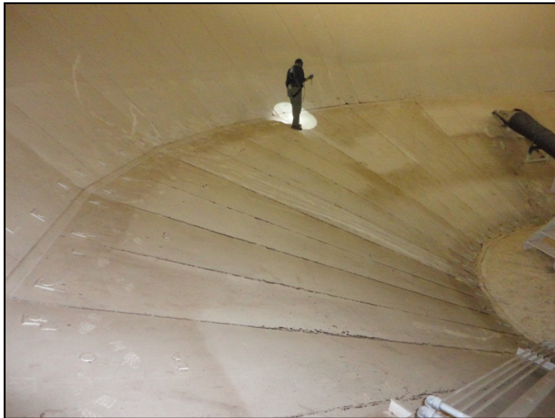
Inspection of bottom of emptied and cleaned tank
