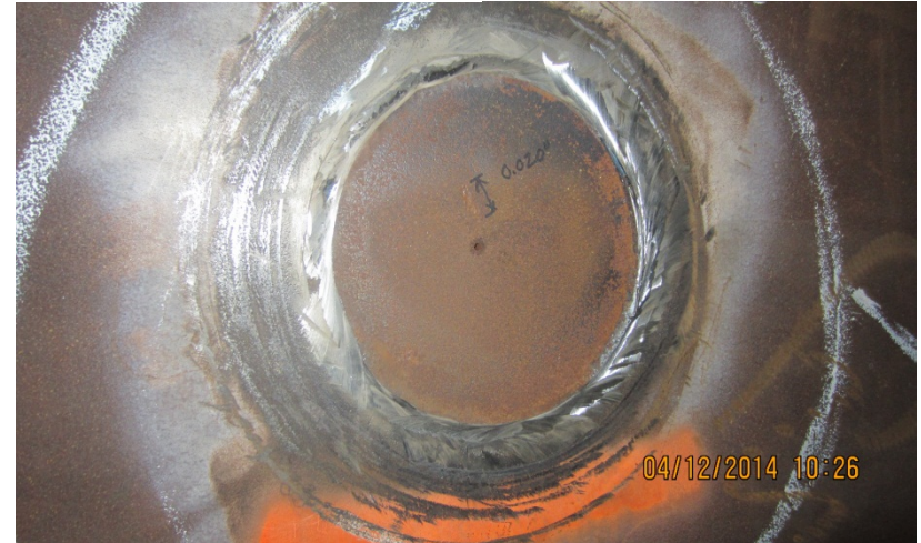
Location of repair with patch removed
