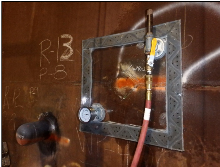
Vacuum box testing conducted at identified location
