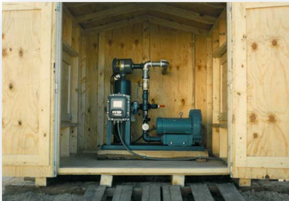
Typical air pump system
