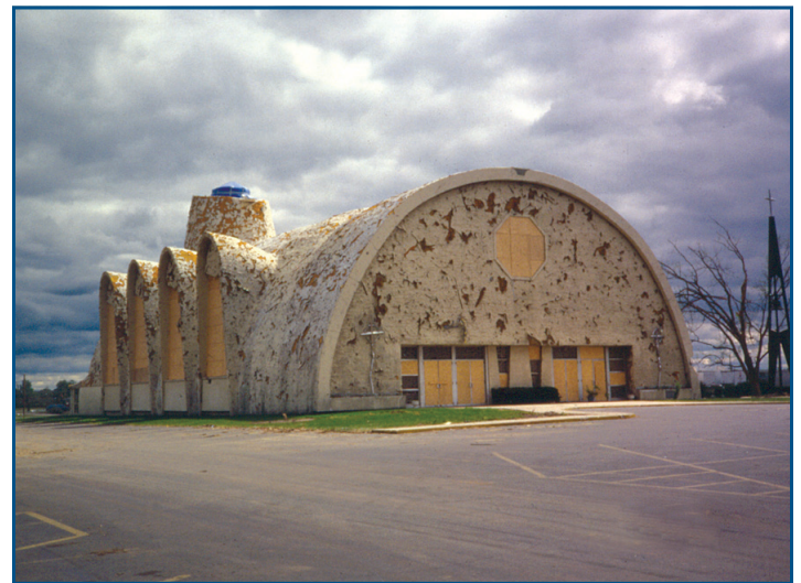
Figure 6: Although struck by a strong tornado, the SPF roof system of this Plainfield, IL, building did not blow off (1990 Tornado)
