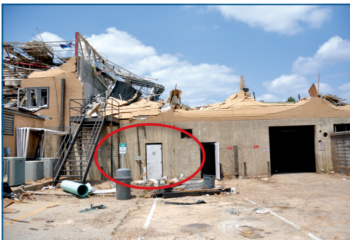
Figure 9: An EOC in Tuscaloosa, AL, that remained intact even though the story above it collapsed (Tornado 2011)
